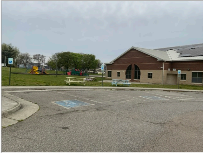
OVERVIEW OF ACCESSIBLE PARKING AREA
