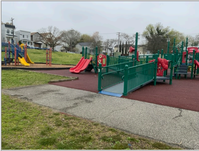
ACCESSIBLE ROUTE TO PLAYGROUND
