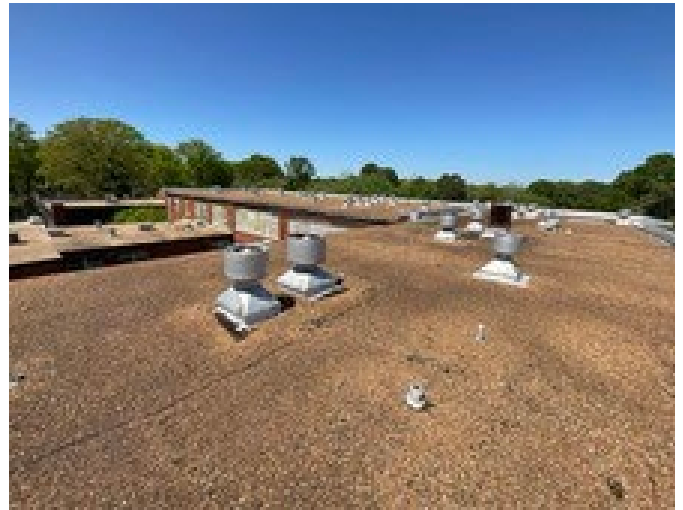
8 - MAIN ROOF OVERVIEW
