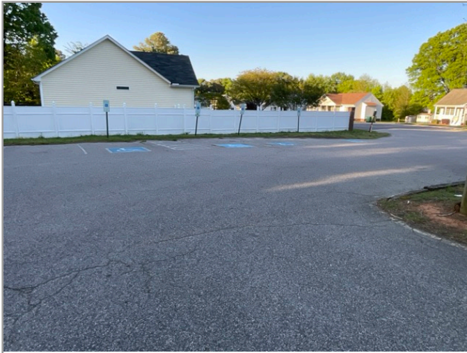
OVERVIEW OF ACCESSIBLE PARKING AREA
