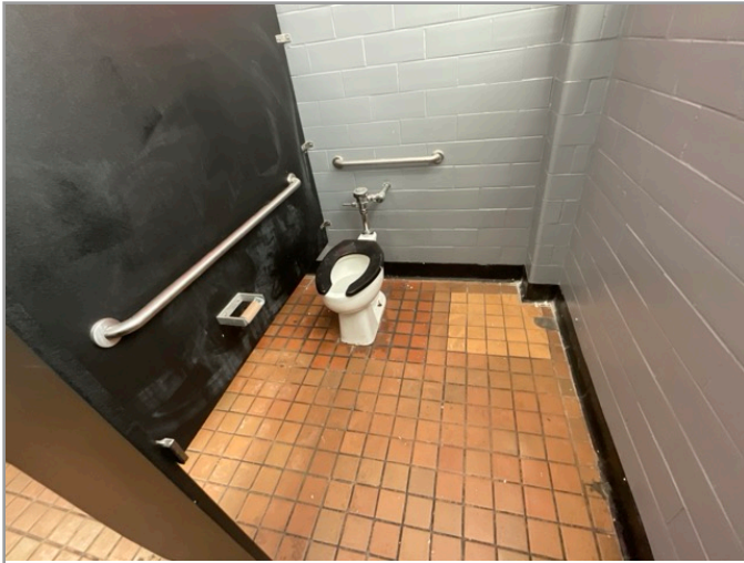
TOILET STALL OVERVIEW
