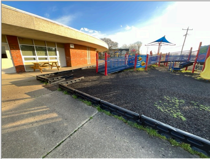
ACCESSIBLE ROUTE TO PLAYGROUND
