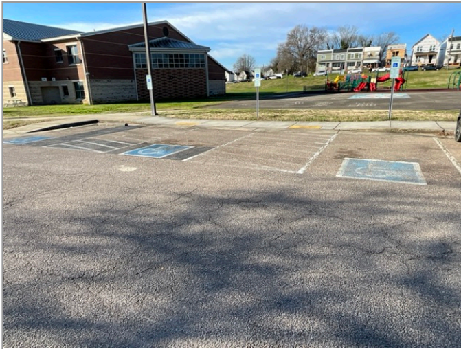
OVERVIEW OF ACCESSIBLE PARKING AREA
