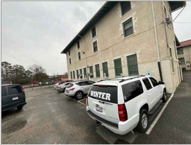
OVERVIEW OF ACCESSIBLE PARKING AREA
