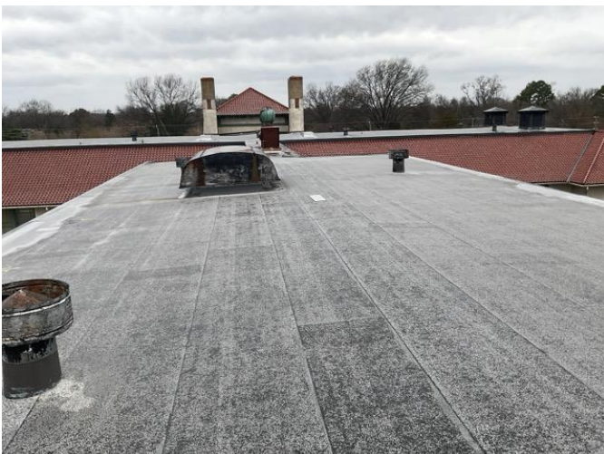
5 MODIFIED BITUMEN ROOF
