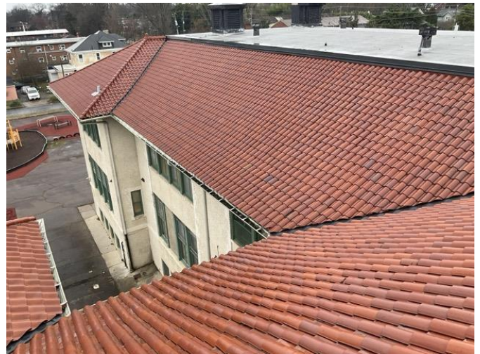
4 - SPANISH TILE ROOF
