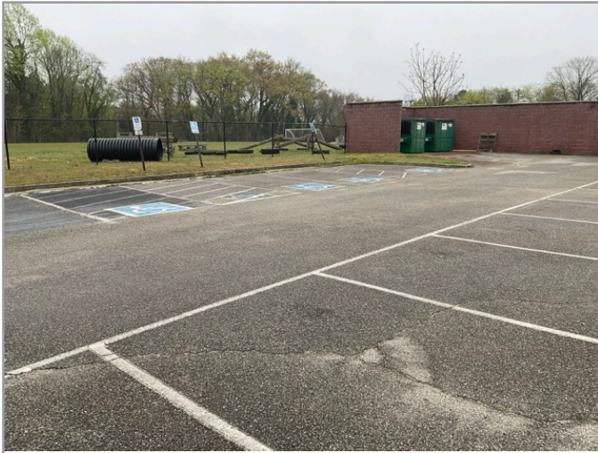
OVERVIEW OF ACCESSIBLE PARKING AREA
