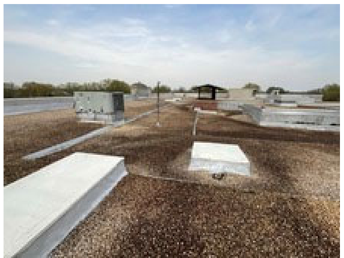
6 - MAIN ROOF OVERVIEW
