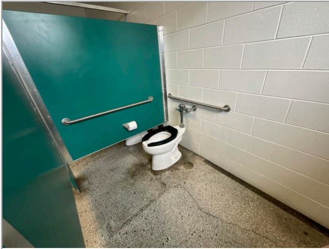
TOILET STALL OVERVIEW
