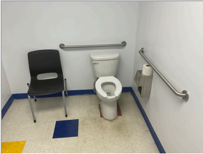
TOILET STALL OVERVIEW
