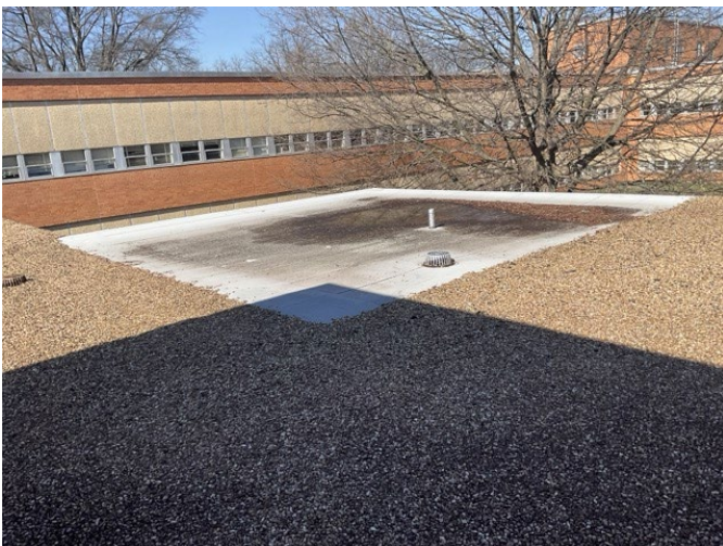
5 - MODIFIED BITUMEN ROOF
