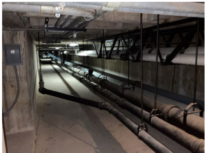
12 - PLUMBING AND HVAC PIPE TUNNELS
