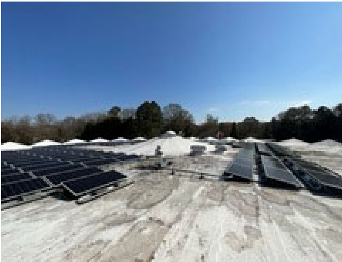
7 - ADDITIONAL ROOF OVERVIEW
