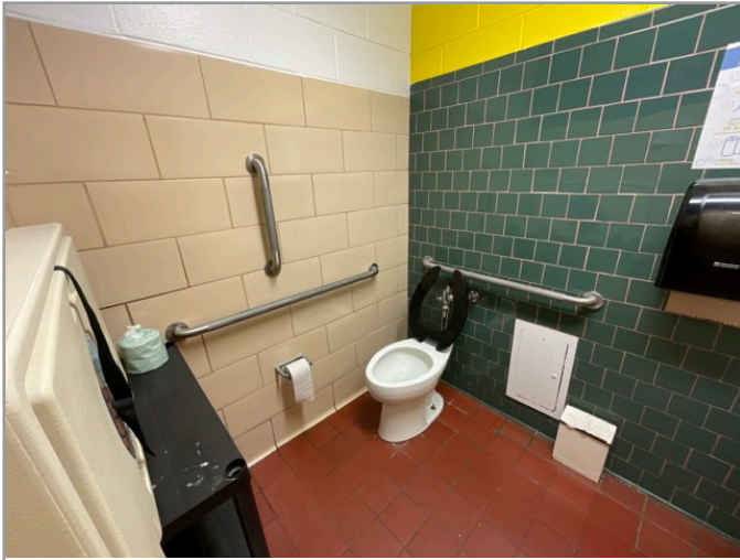
TOILET STALL OVERVIEW
