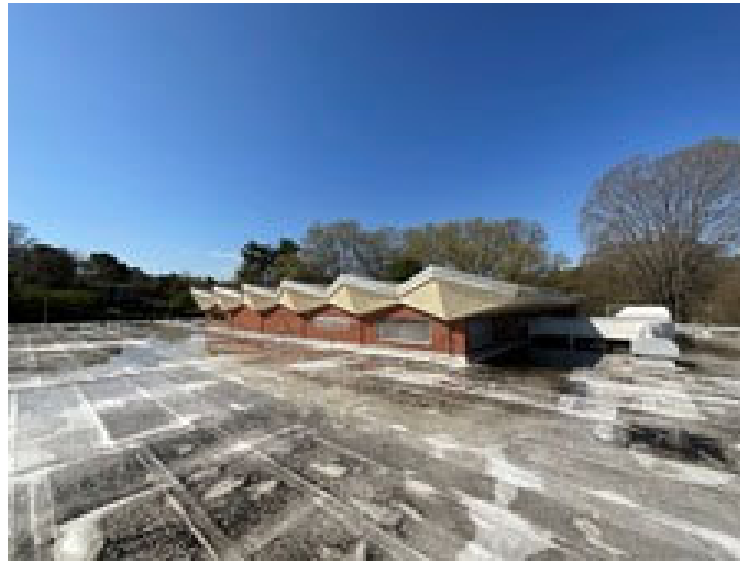
8 - CAFETORIUM ROOF OVERVIEW
