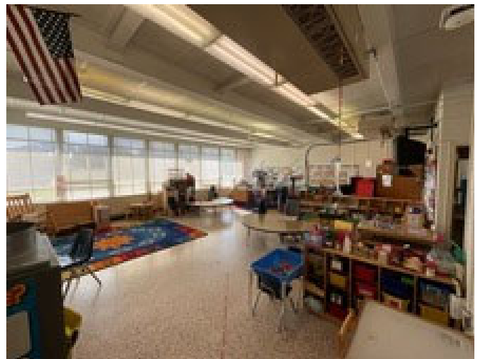
18 - TYPICAL CLASSROOM WITH TERRAZZO
