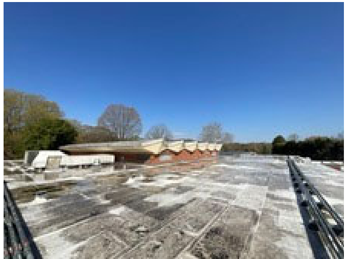
6 - FLUID APPLIED ROOF OVERVIEW
