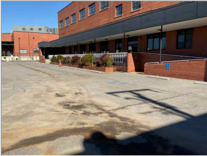
OVERVIEW OF ACCESSIBLE PARKING AREA
