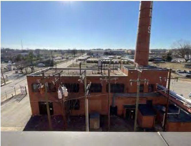
7 - FIRE PUMP BUILDING ROOF
