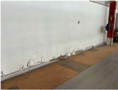
Concrete is degraded and spalled - AssetCALC ID: 7350915
