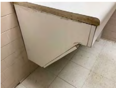
Delaminating - AssetCALC ID: 7350866
