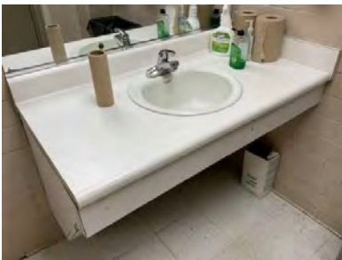
Delaminating - AssetCALC ID: 7350902
