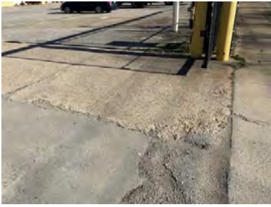
Concrete is degraded and spalled - AssetCALC ID: 7350915
