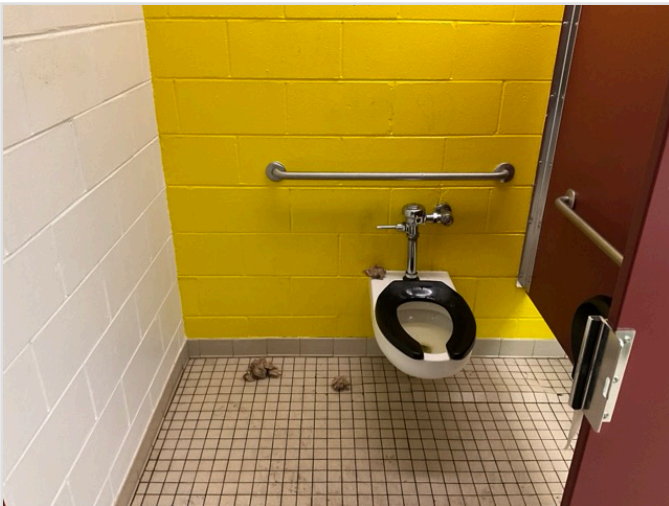
TOILET STALL OVERVIEW
