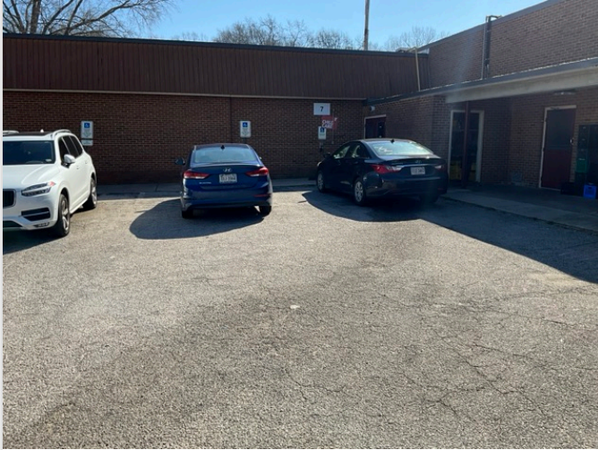
OVERVIEW OF ACCESSIBLE PARKING AREA
