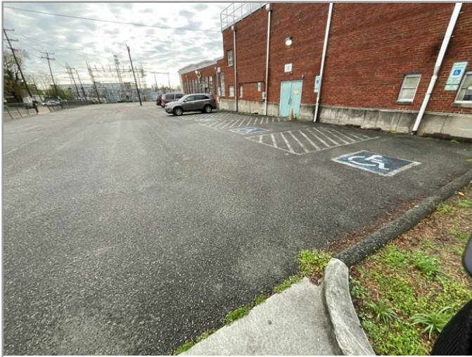
OVERVIEW OF ACCESSIBLE PARKING AREA
