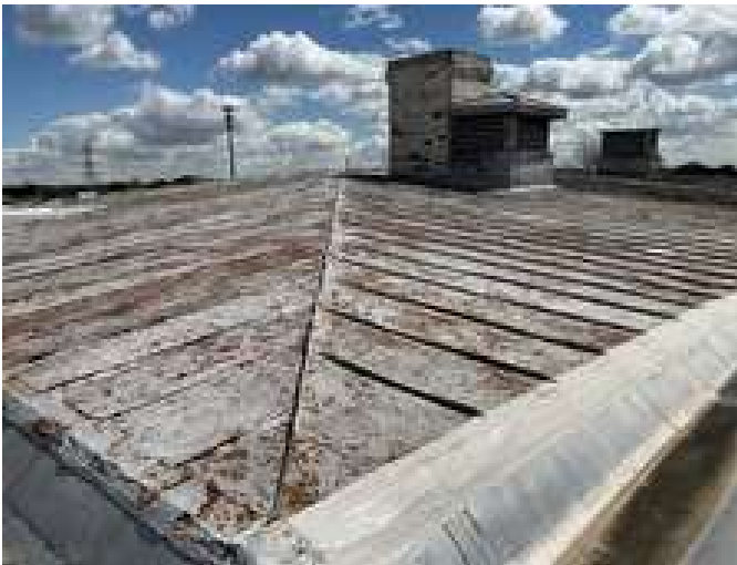
3 - MAIN ROOF OVERVIEW
