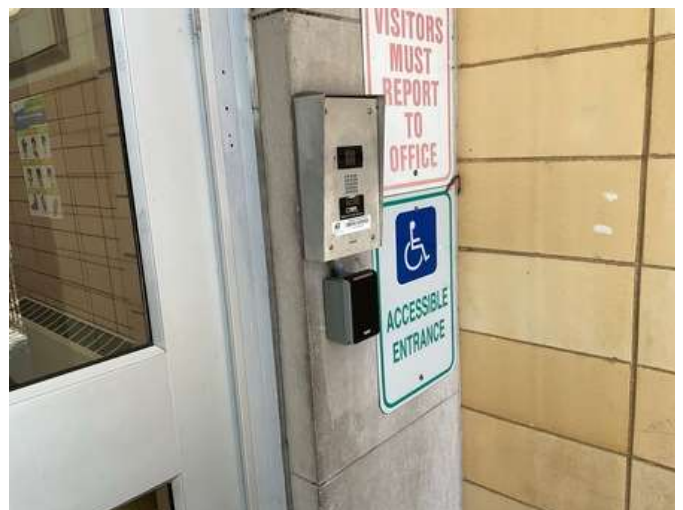
24 - INTERCOM AND BUILDING ACCESS
