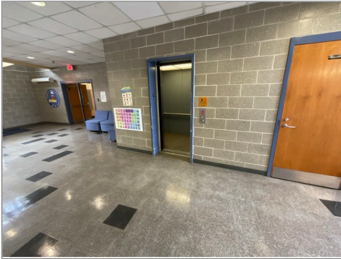
LOBBY LOOKING AT CABS (WITH DOORS OPEN)
