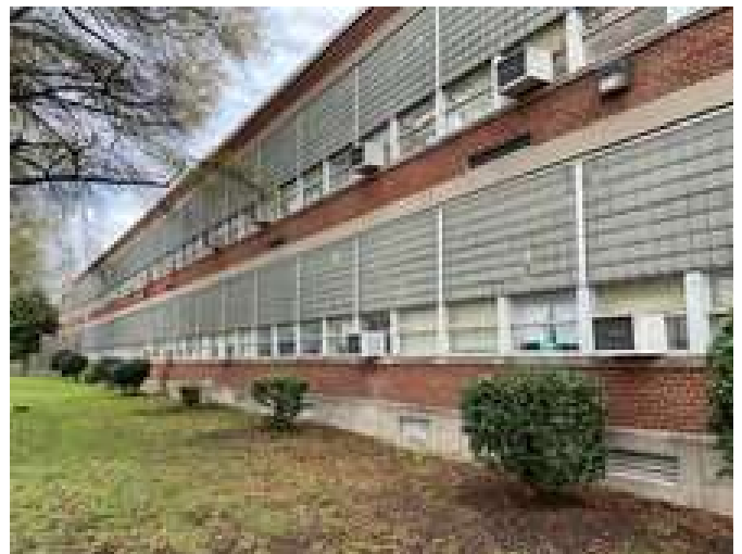
6 - GLASS BLOCK FACADE
