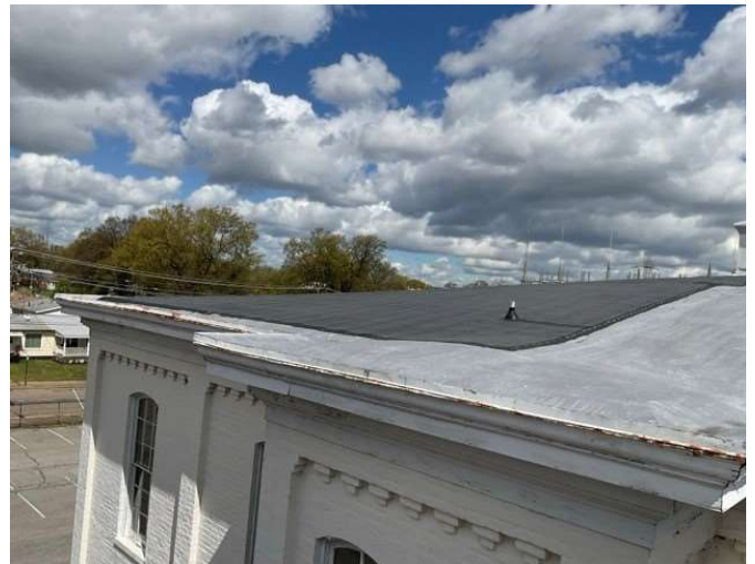
4 - SECONDARY ROOF OVERVIEW
