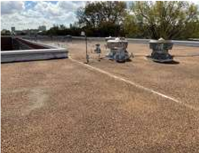
7 - PRIMARY ROOF OVERVIEW
