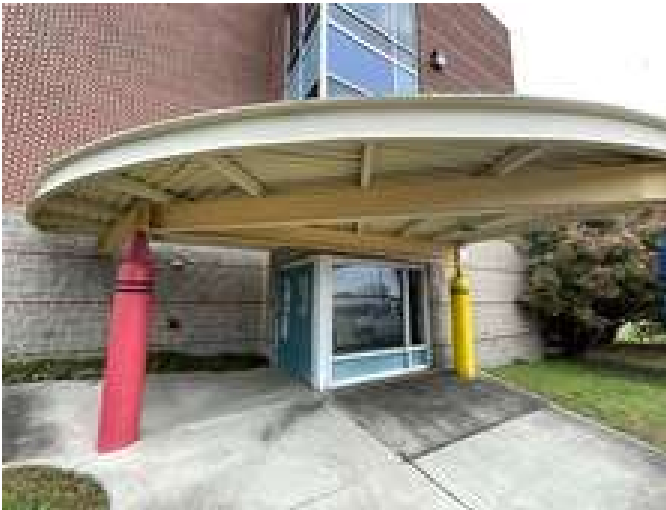
7 - ROOF STRUCTURE SIDE ENTRANCE
