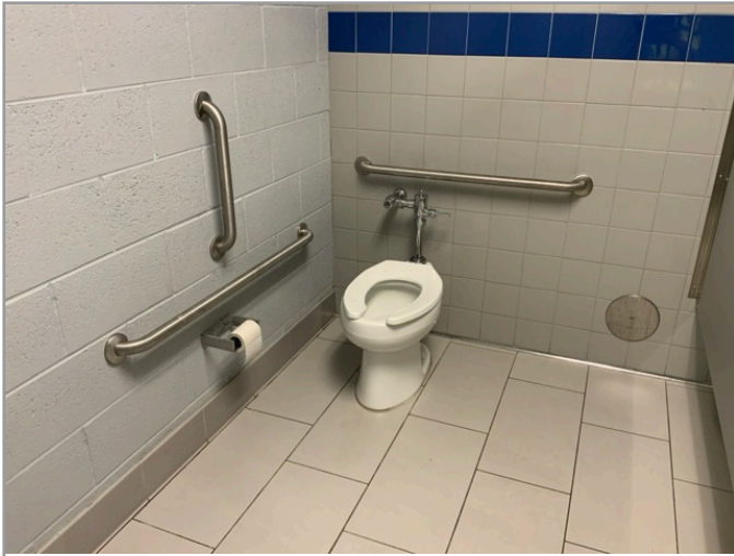
TOILET STALL OVERVIEW
