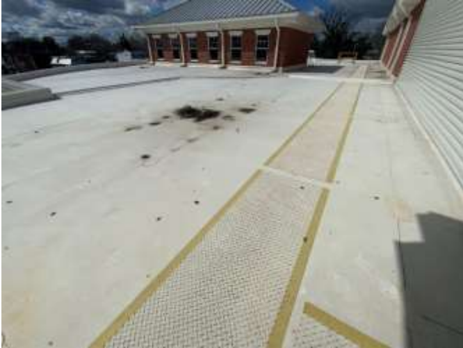
5 – SINGLE PLY ROOF
