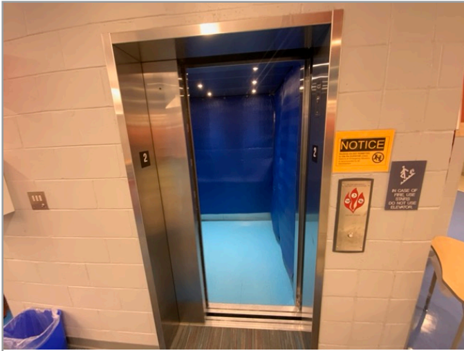
LOBBY LOOKING AT CABS
