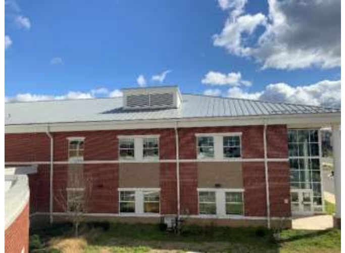
6 – ROOF OVERVIEW METAL ROOF
