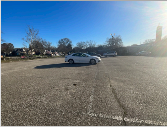
OVERVIEW OF ACCESSIBLE PARKING AREA
