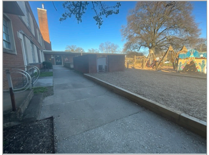
ACCESSIBLE ROUTE TO PLAYGROUND
