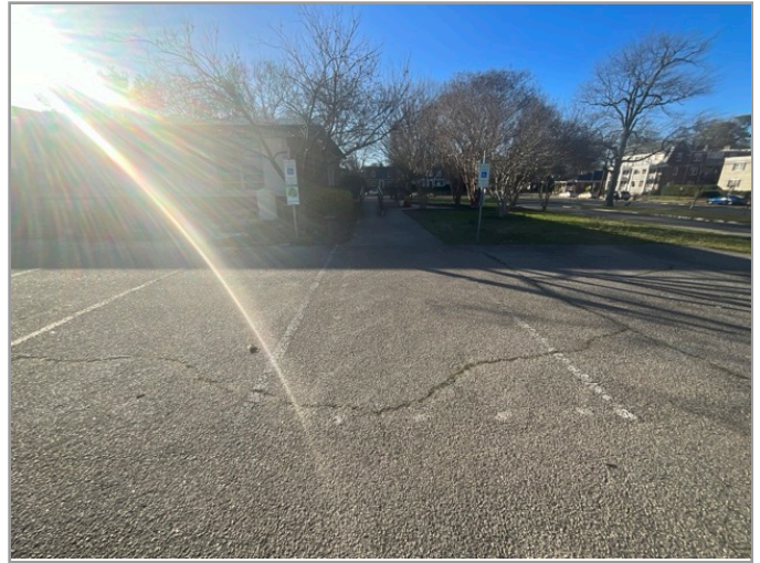
OVERVIEW OF ACCESSIBLE PARKING AREA
