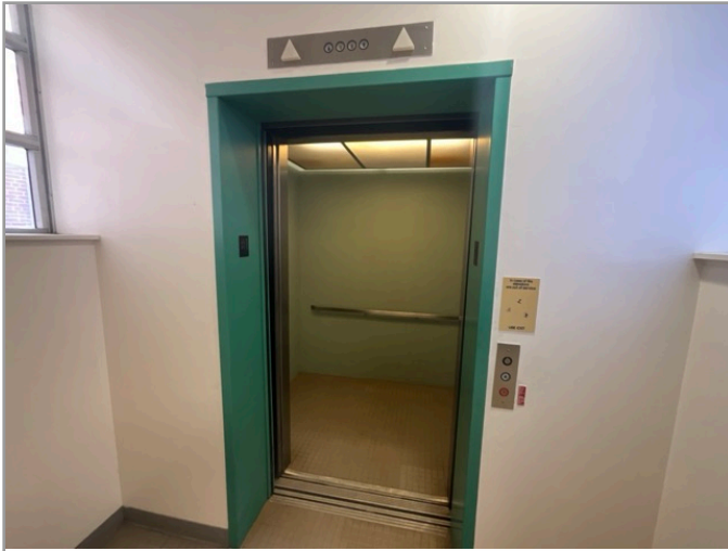
LOBBY LOOKING AT CABS
