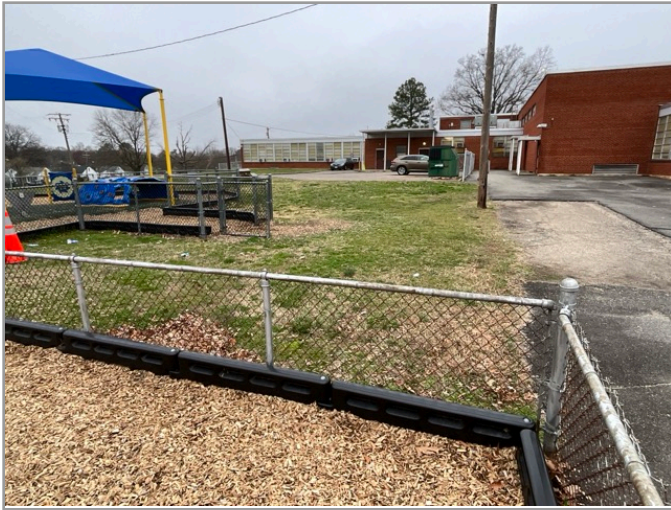
ACCESSIBLE ROUTE TO PLAYGROUND
