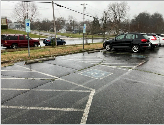
OVERVIEW OF ACCESSIBLE PARKING AREA
