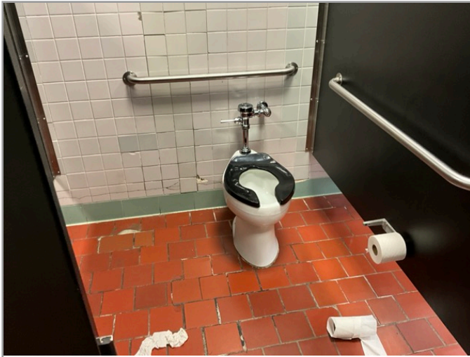
TOILET STALL OVERVIEW
