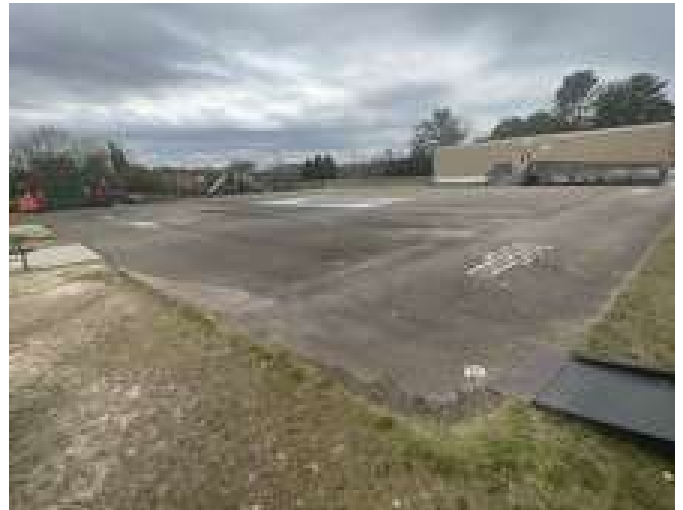
8 - ASPHALT PLAY SURFACE
