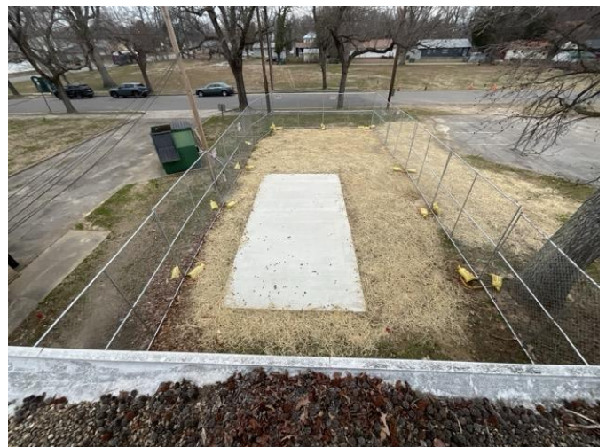
6 - COOLING PLANT TO BE INSTALLED
