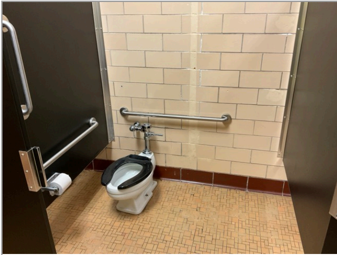
TOILET STALL OVERVIEW
