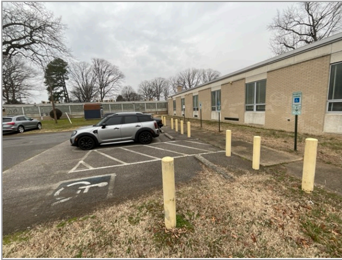
OVERVIEW OF ACCESSIBLE PARKING AREA
