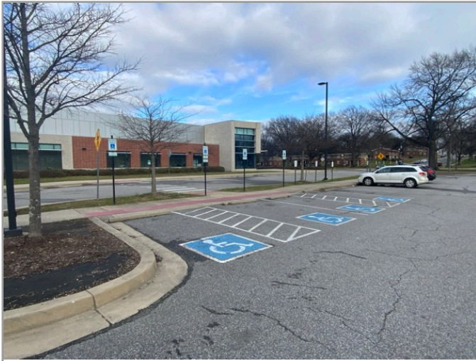
OVERVIEW OF ACCESSIBLE PARKING AREA
