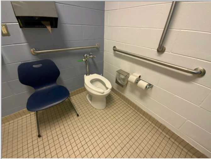
TOILET STALL OVERVIEW
