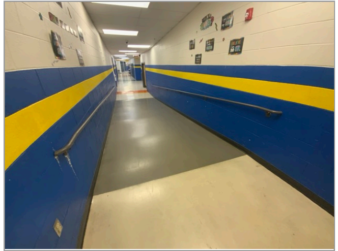
ACCESSIBLE INTERIOR RAMP
