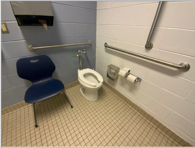
TOILET STALL OVERVIEW
