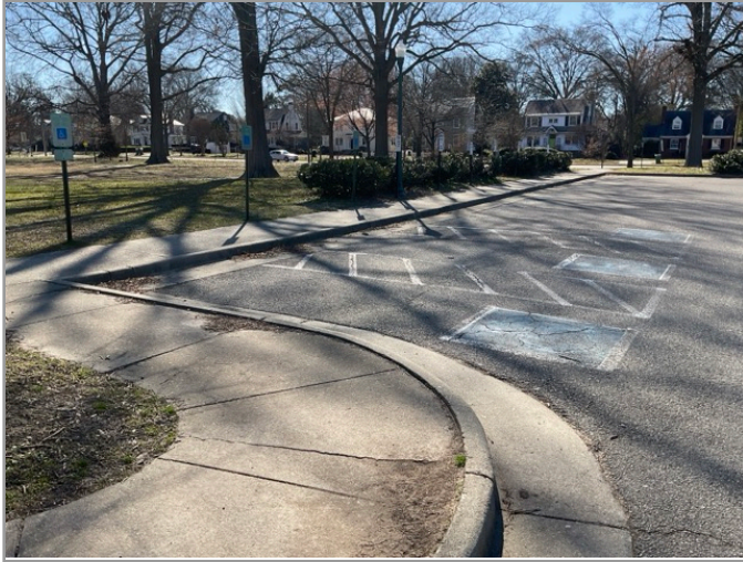
OVERVIEW OF ACCESSIBLE PARKING AREA
