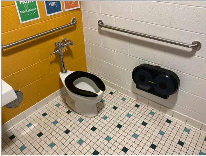
TOILET STALL OVERVIEW
