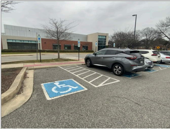
OVERVIEW OF ACCESSIBLE PARKING AREA
