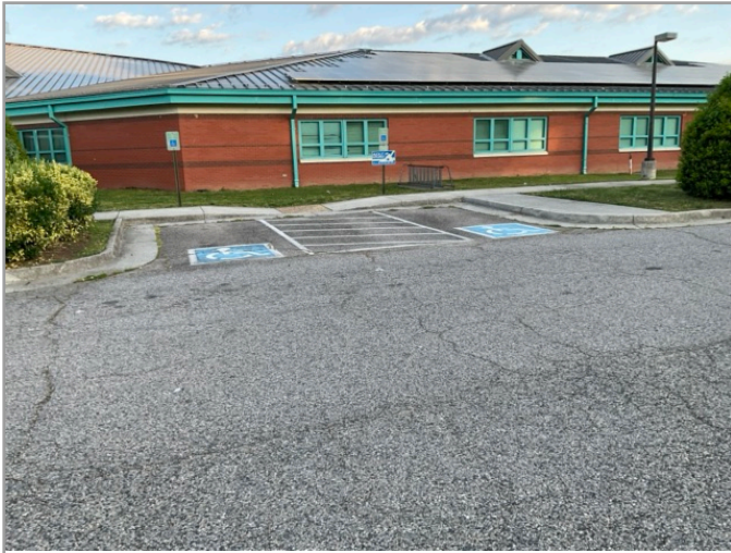
OVERVIEW OF ACCESSIBLE PARKING AREA
