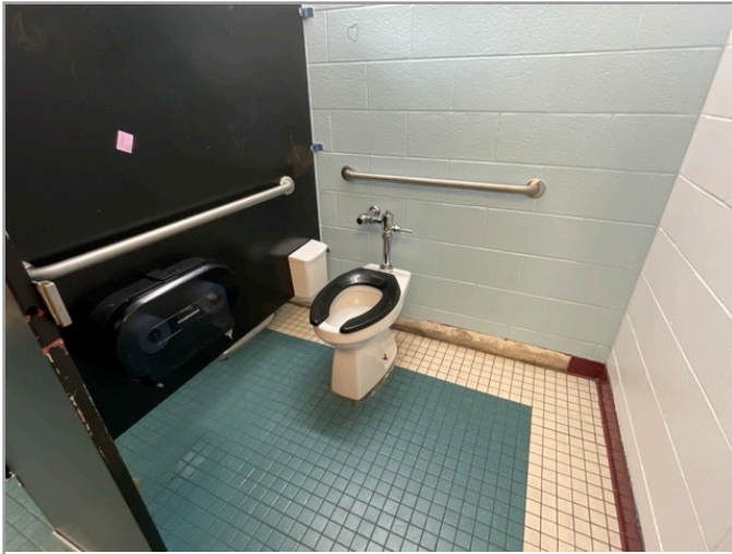
TOILET STALL OVERVIEW
