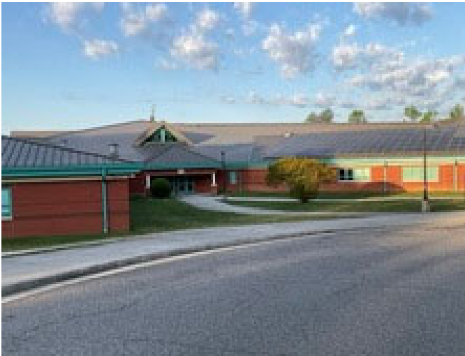
7 - PRIMARY ROOF OVERVIEW
