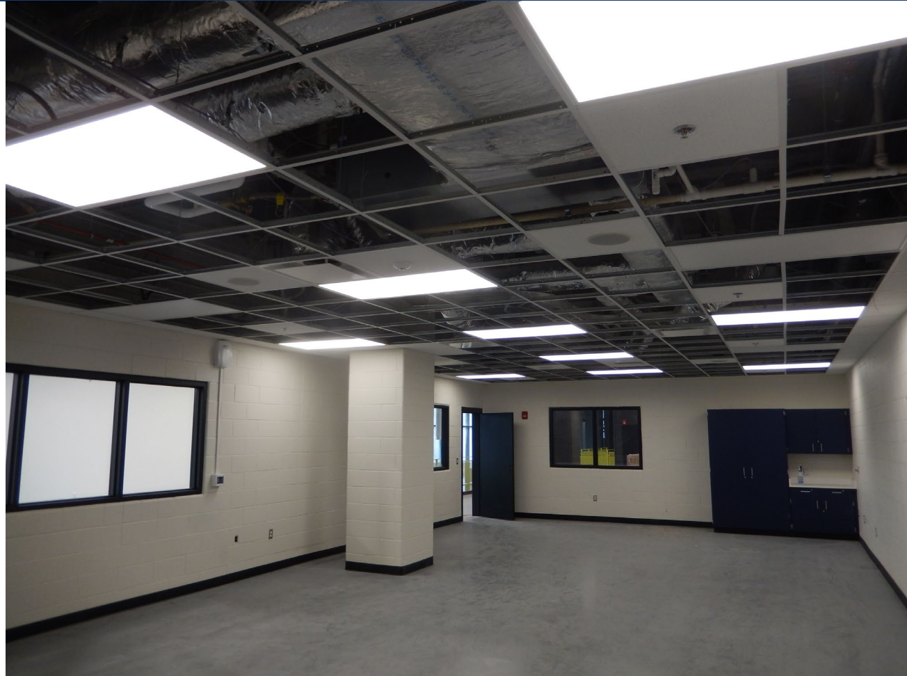
Level 2 ceiling grid and lights
