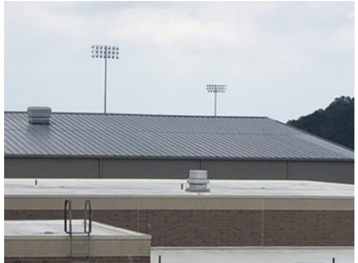
Standing Seam Metal Roofing
