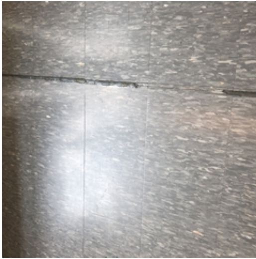
Damaged VCT
