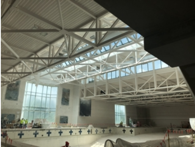
Roof Deck / Girders
