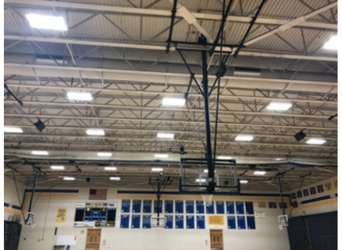
Roof Deck / Joist Framing
