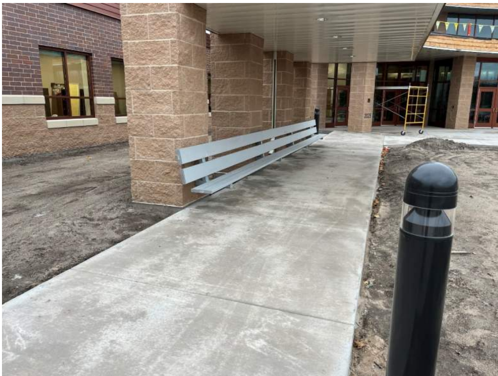
Exterior Site Improvements at Radius Entry
