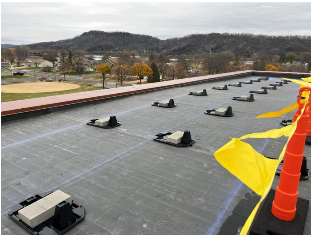
Solar Connections – Ballasts and Pedestals for Solar Panels Installed
