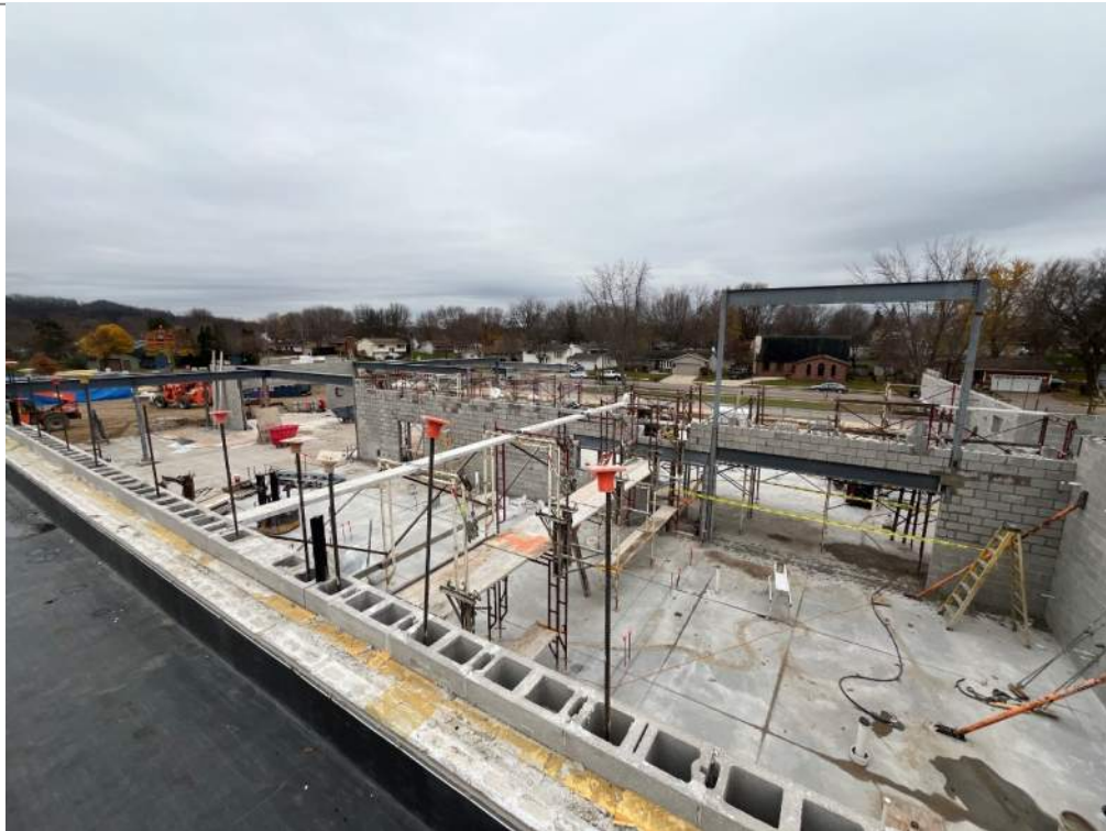
Segment F Classroom Addition CMU Bearing Walls in-Progress
