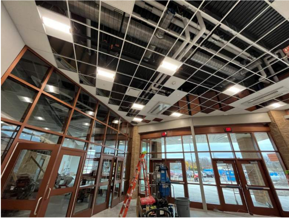
Segment D Radius Entry – Final Finishes
