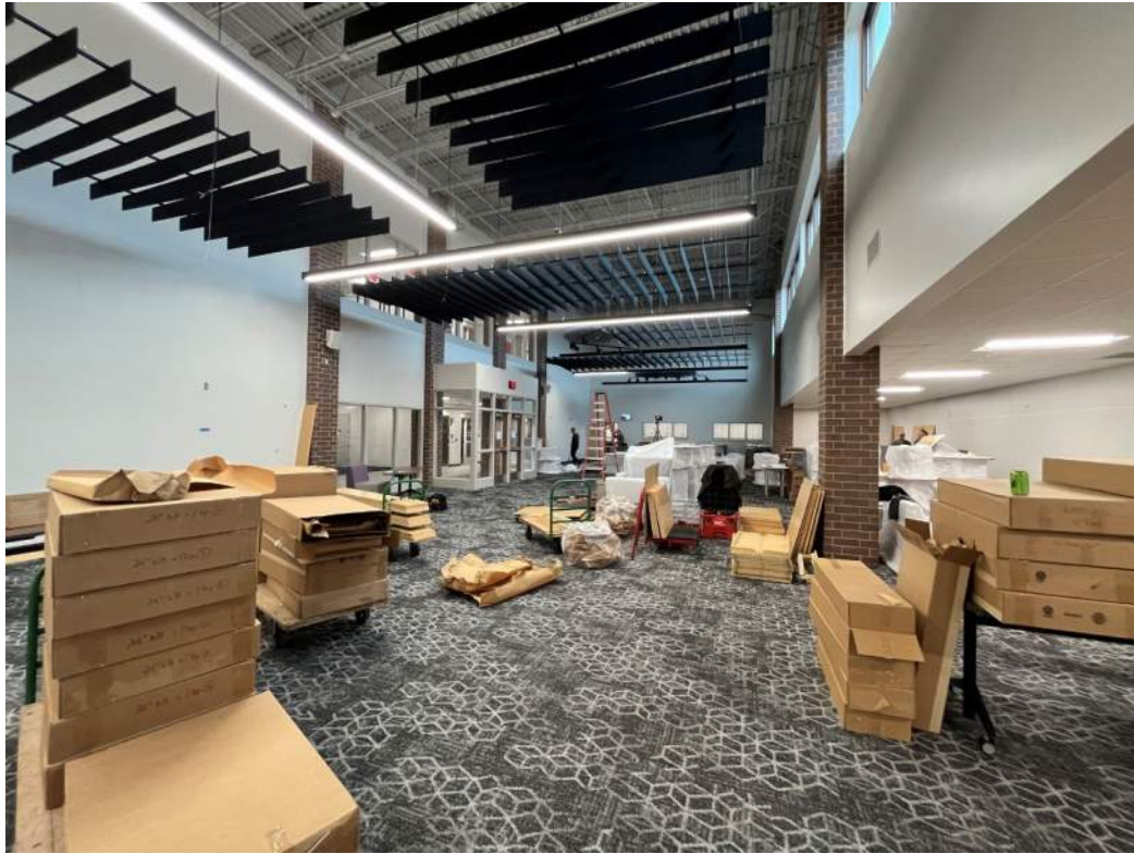
Segment E/F – LMC Furniture and Bookcase Installation In-Progress
