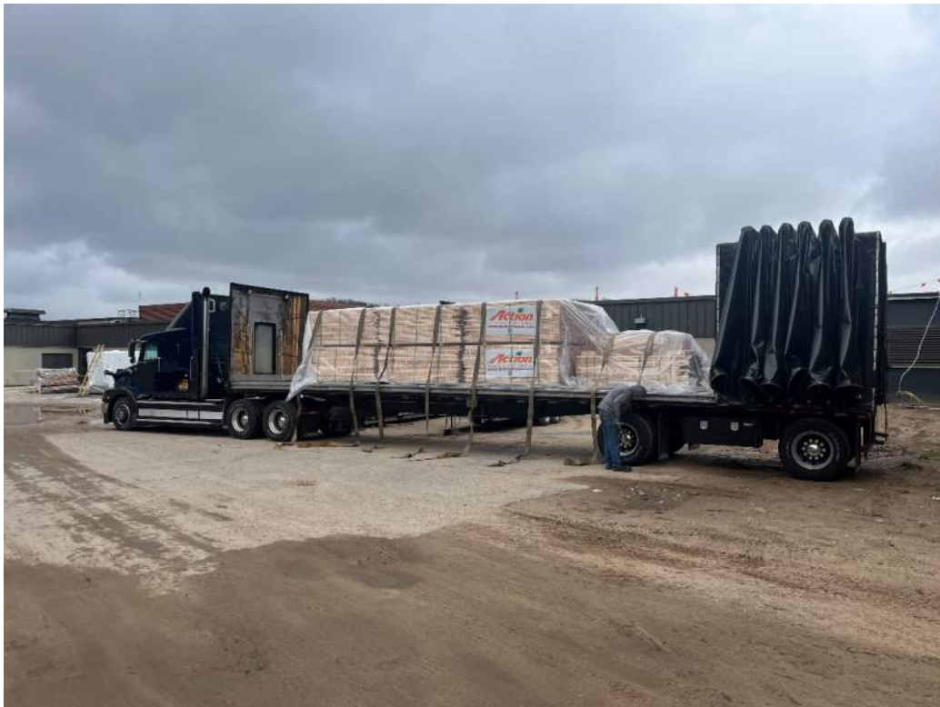
GYM 194 Wood Floor Delivered
