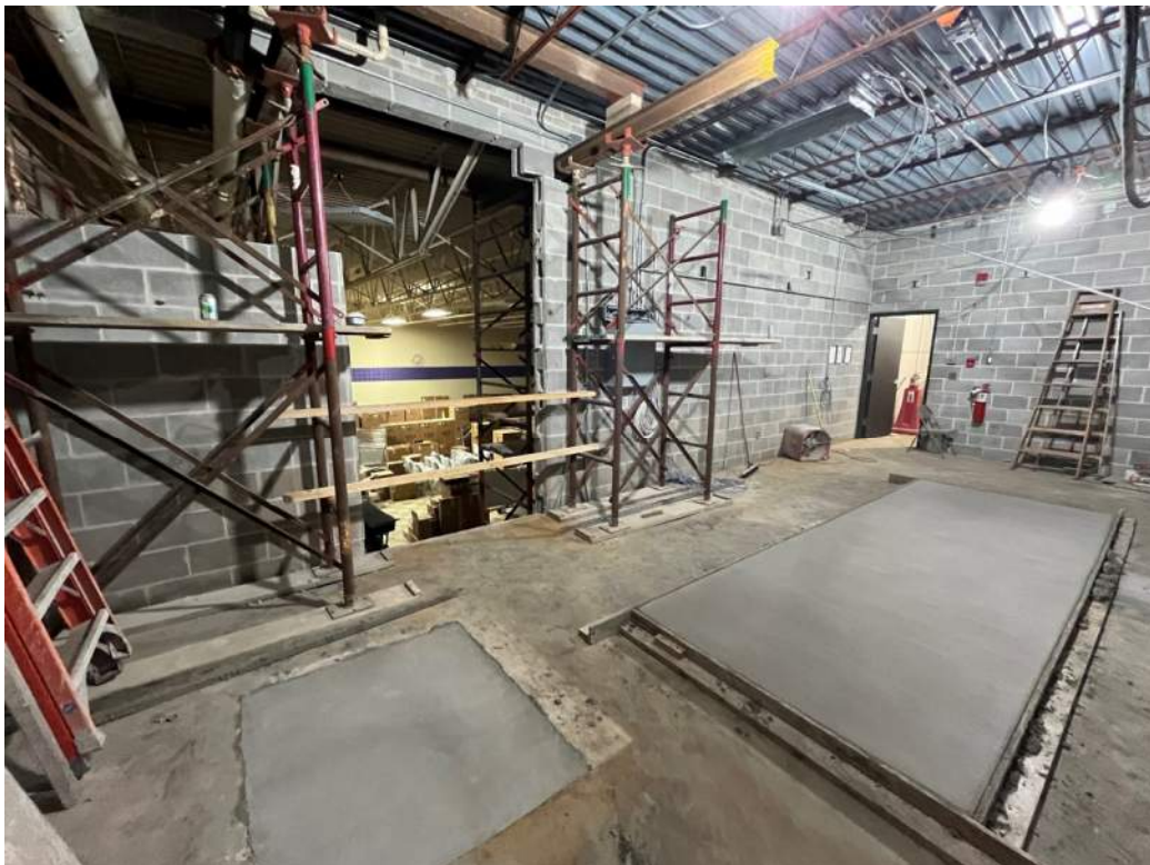
Segment A Mechanical Mezzanine – Equipment Pads Poured
