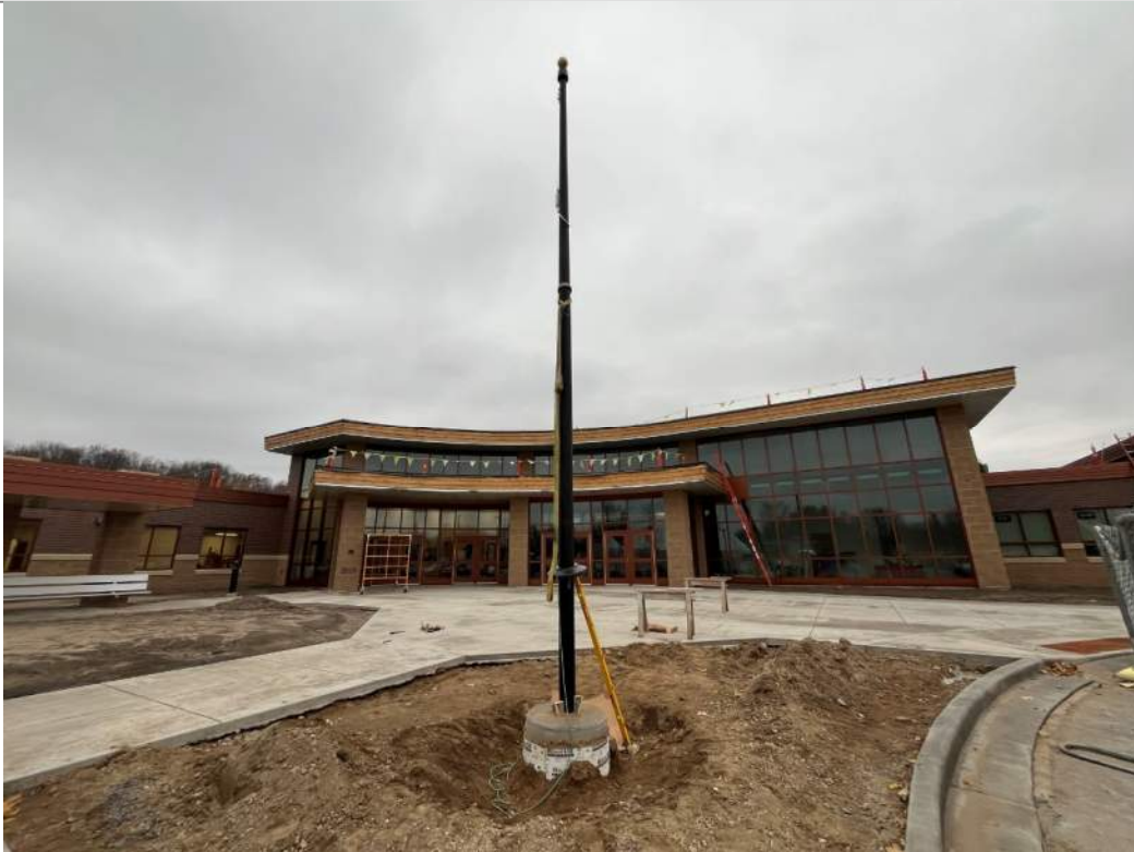
Segment D Radius Entry – Flag Pole Installed
