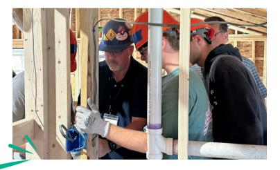
In September, the students began roughing in the wiring to accomodate an extensive machine shop, wood shop, conference room, and showroom. They'll continue the project with installation of electrical finishes including light fixtures and receptacles. This also includes surface mounting, conduit, and light fixtures to reflect an industrial style for the antique equipment showroom.
