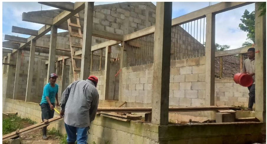
Construction continues on a school made of cinder blocks and cements, a great improvement for the students in Rio Blanco.
