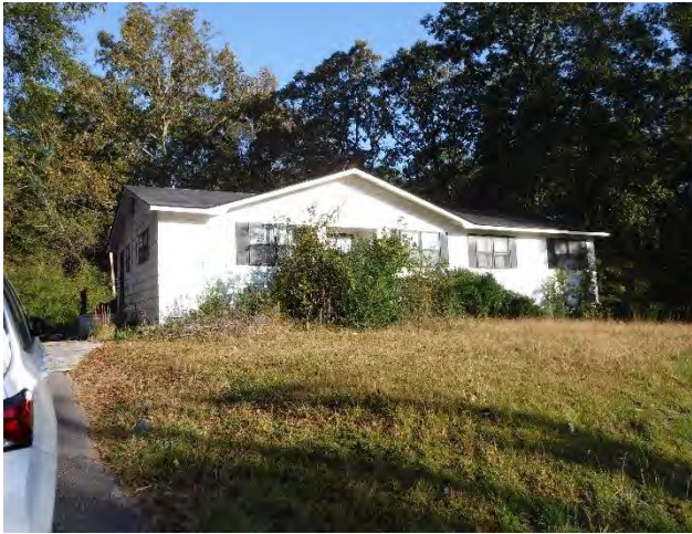
Photo 13: Typical view north of eastern adjoining residential development.
