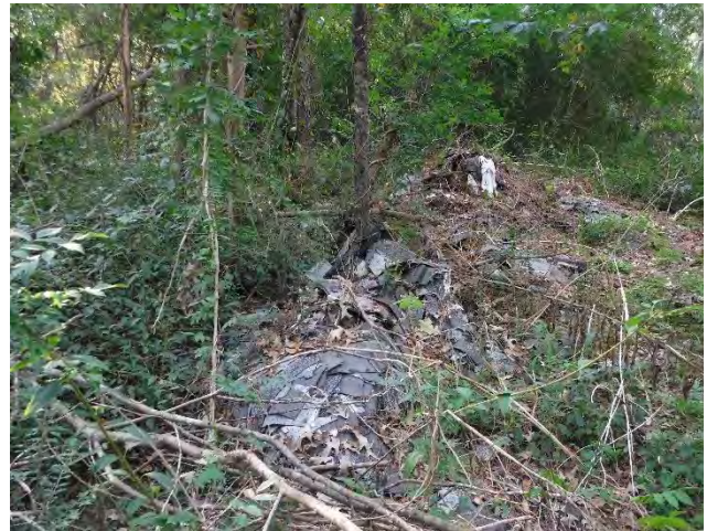
Photo 6: Typical view of construction materials and debris on Site.
