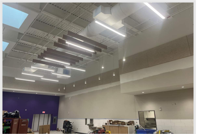
Bottom Right: a view of the finished ceiling in the Commons with as the acoustical baffles are hung around the new light fixtures
