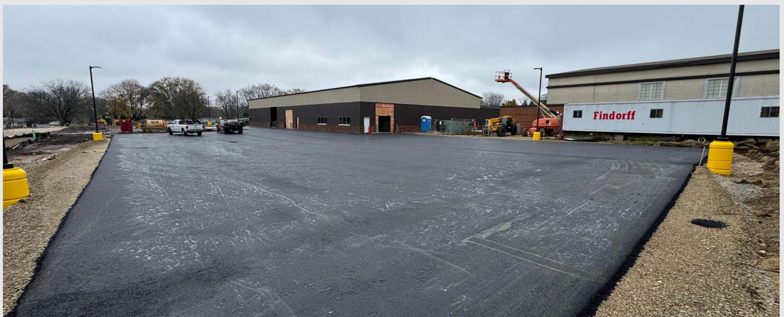
Below: a photo from earlier this week following installation of the asphalt binder course at the Yahara Site
