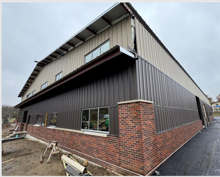
Top Left: a photo of the Maintenance Building exterior high lighting the brick and metal panel enclosure
