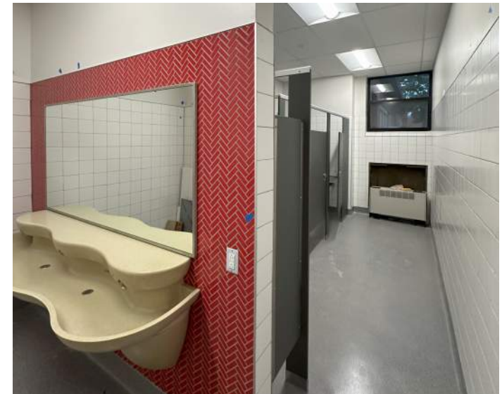
Ridgeview - Level 2 Restroom
