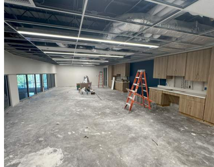
1964 (Area A) Progress
