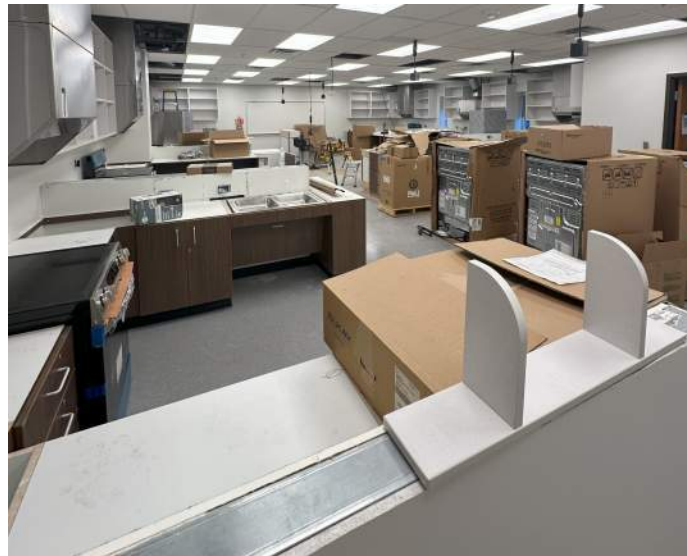
Progress 100's Wing
