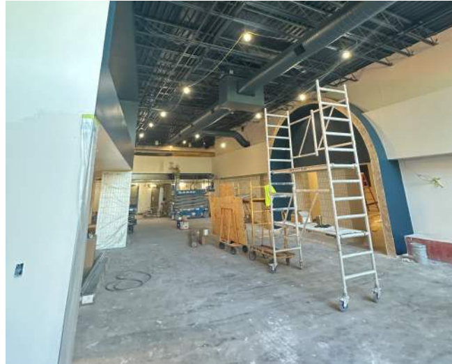
1964 (Area A) Progress
