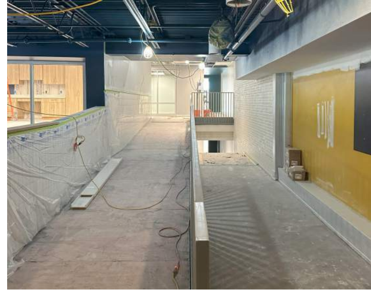
1964 (Area A) Progress
