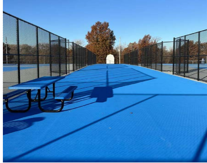
Center Spectator Concourse Looking West
