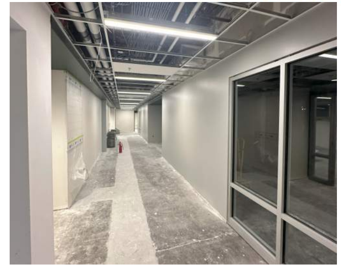
1964 (Area A) Progress
