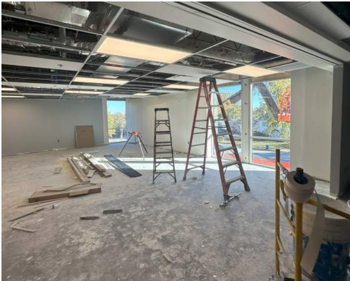
1964 (Area A) Progress
