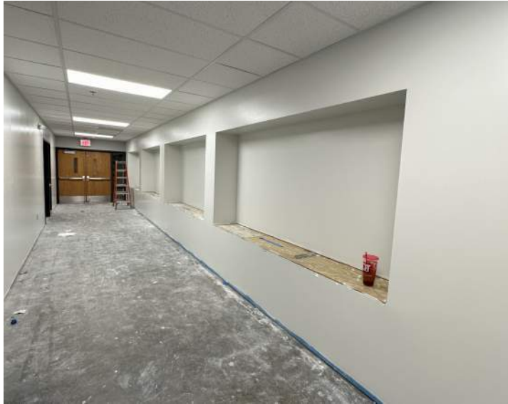
Progress 100's Wing
