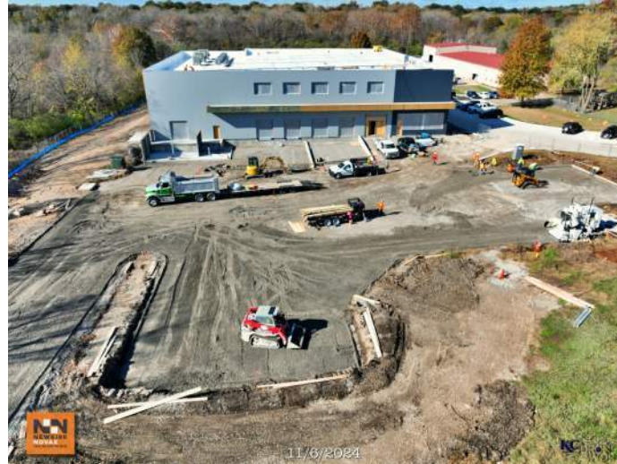
East Lot Construction
