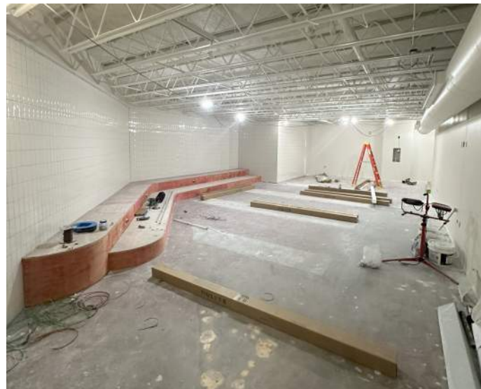
1964 (Area A) Progress
