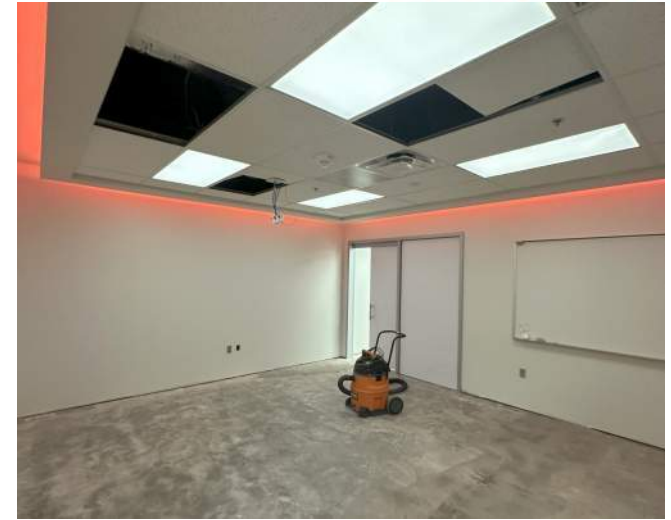
Progress 100's Wing
