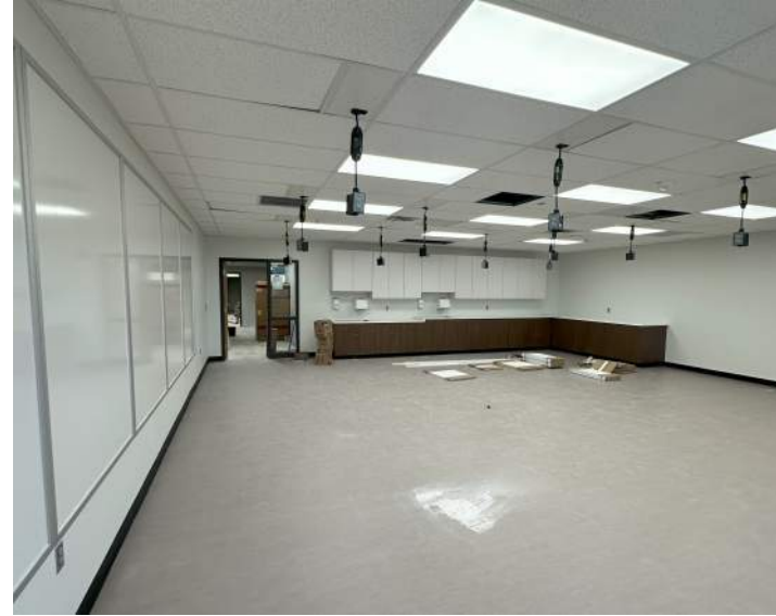
Progress 100's Wing
