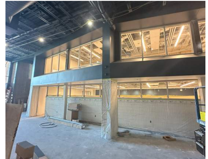
1964 (Area A) Progress
