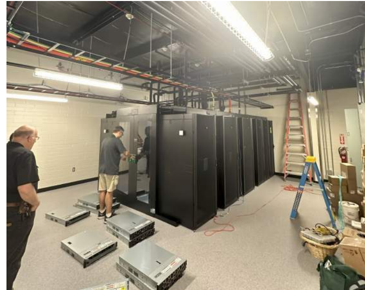
Data Pod Install
