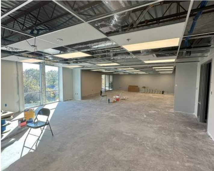
1964 (Area A) Progress
