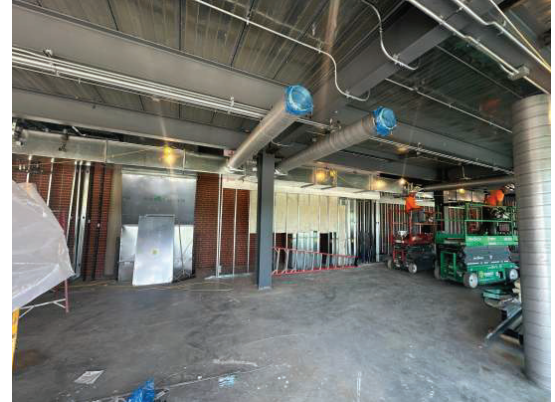
Main Level Ductwork
