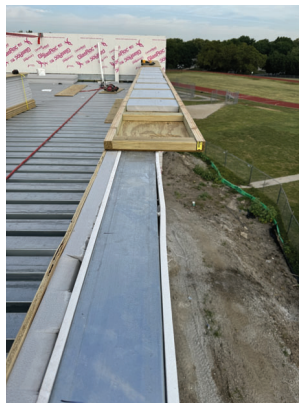
Roof Parapet Blocking
