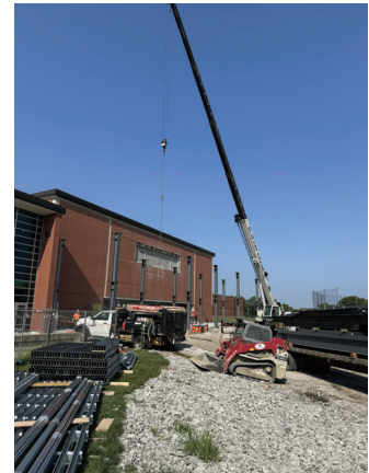
Building Addition Set Columns
