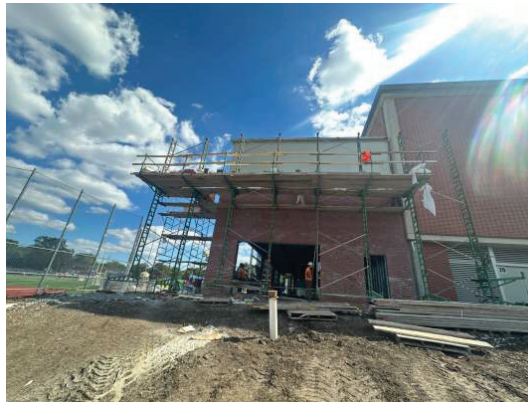
East Wall Brick Install
