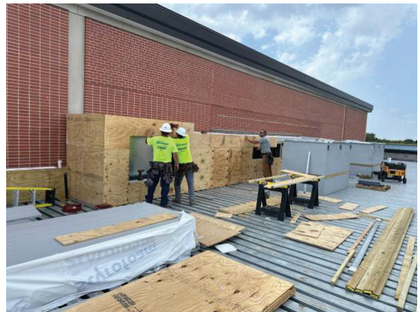
Roof Dog House Wood Blocking
