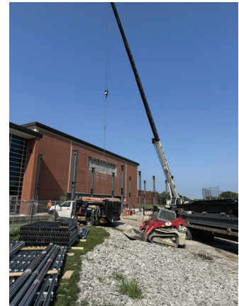
Building Addition Set Columns
