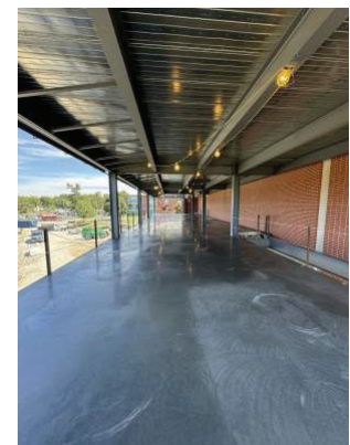
Addition Slab on Deck
