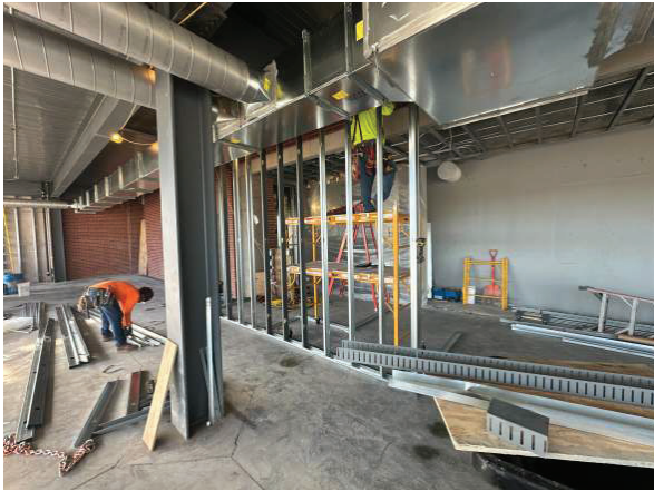
Interior Wall Framing
