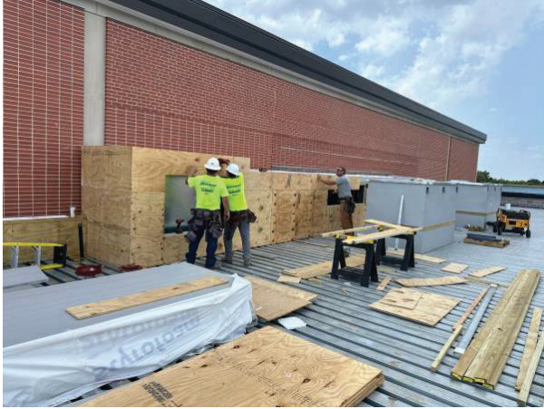
Roof Dog House Wood Blocking
