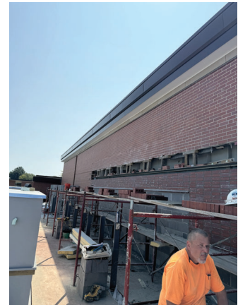
Brick Infill at Roof
