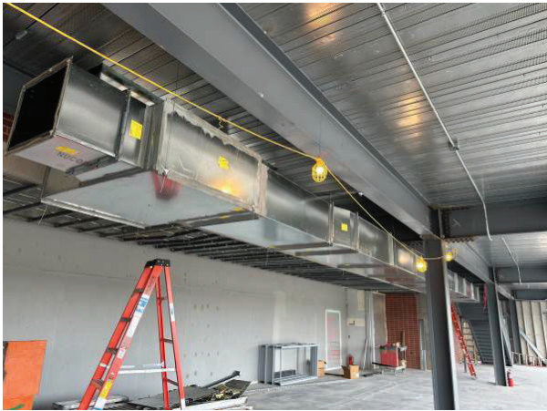
Lower Level Duct Work
