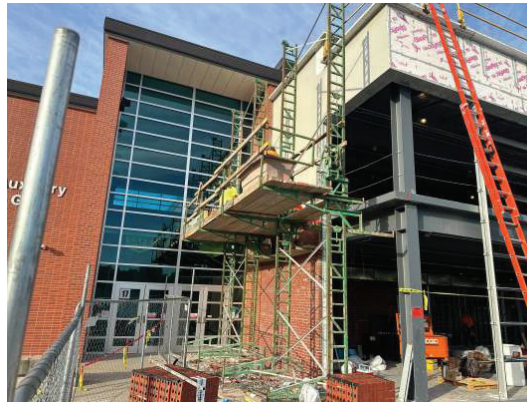
East Wall Brick Install
