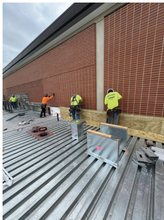
Roof Blocking and Sheathing
