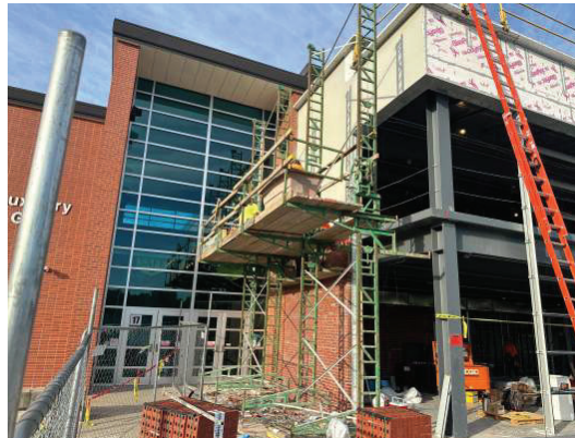
East Wall Brick Install
