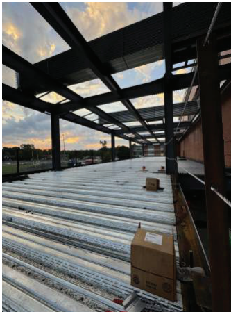
2nd Level Steel Deck
