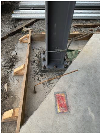
Grout Column Base Plates
