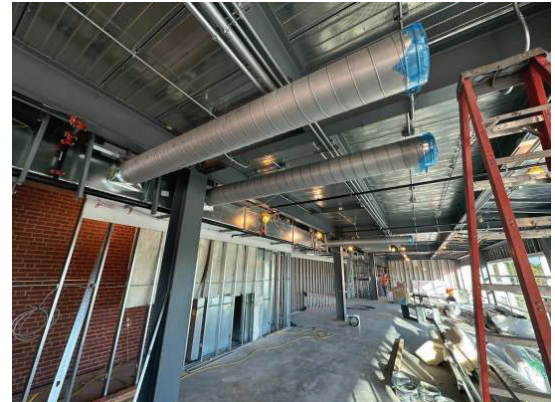
Main Level Ductwork
