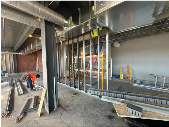
Interior Wall Framing
