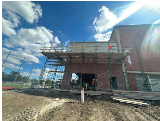
East Wall Brick Install
