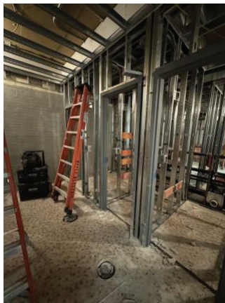
Restroom Wall Framing
