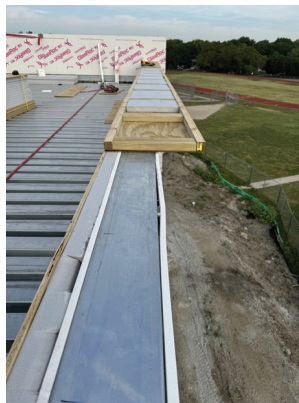
Roof Parapet Blocking
