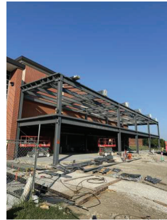
Columns and Beams Set
