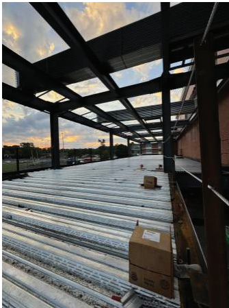
2nd Level Steel Deck
