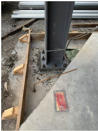
Grout Column Base Plates
