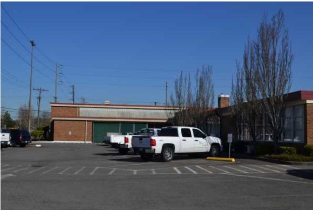
South elevation of original building west wing and west elevation of southern addition, facing north
