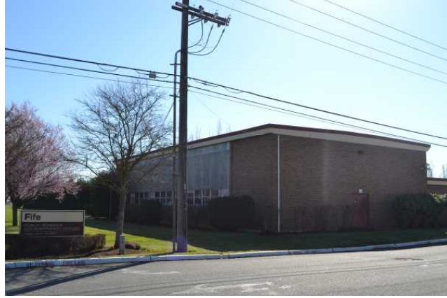
North and west elevations of original building's west projection, facing east
