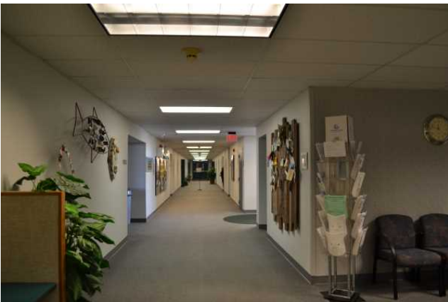
Interior of main building east wing, facing east
