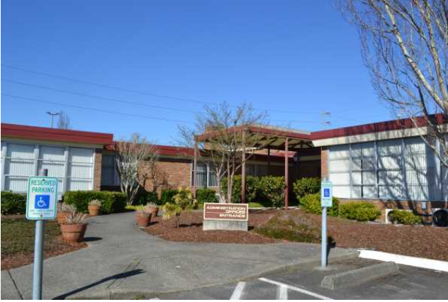
Main entry including original building, covered walkway, and south addition, facing north
