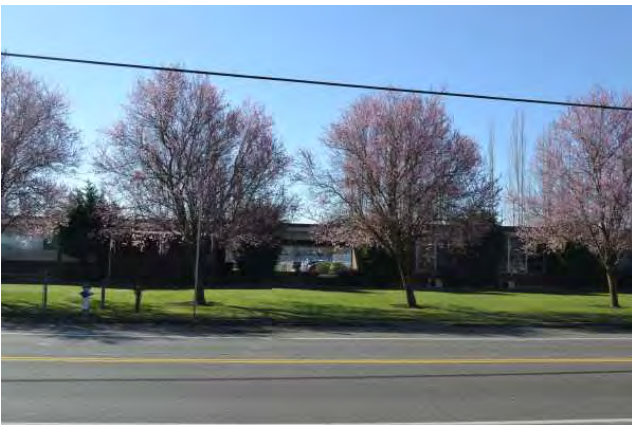
Segment of north elevation, facing south
