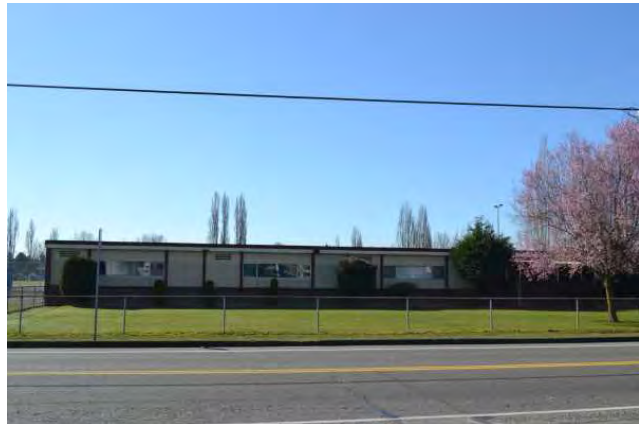
North elevation of east addition, facing south
