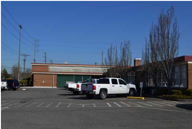
South elevation of original building west wing and west elevation of southern addition, facing north
