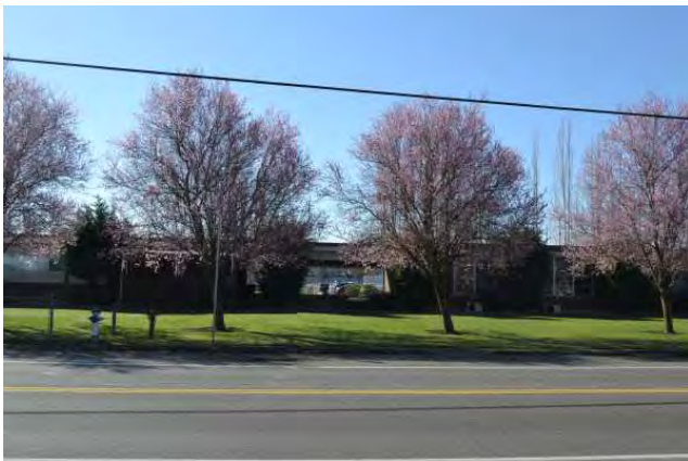
Segment of north elevation, facing south
