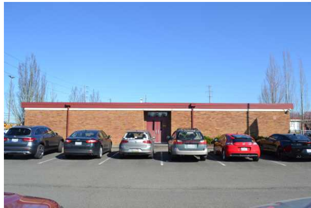
South elevation of southern addition, facing north
