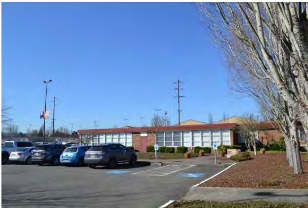
East elevation of south wing addition, facing southwest
