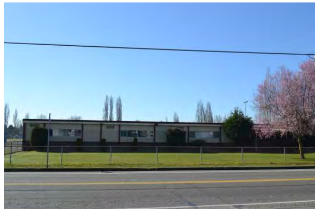
North elevation of east addition, facing south
