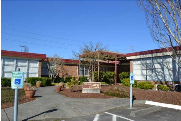
Main entry including original building, covered walkway, and south addition, facing north
