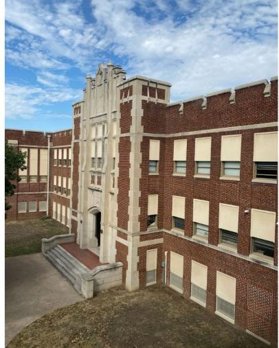
NON-ADA COMPLIANT & UNSECURED MAIN ENTRY AND DAYLIGHTING OBSCURED BY BOARDED WINDOWS
