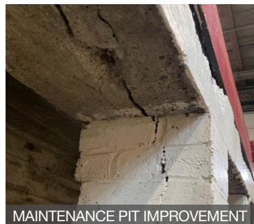
MAINTENANCE PIT IMPROVEMENT
