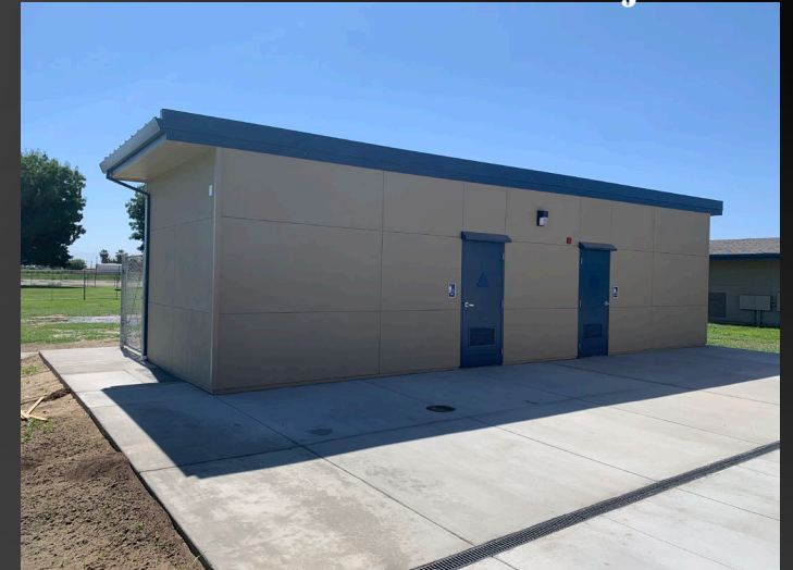
Roosevelt Restroom Project
