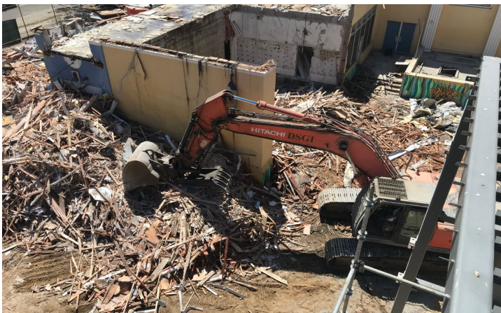
Demolition of old building
