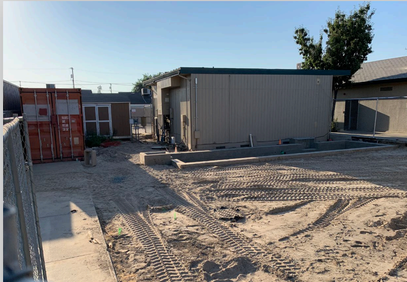
BEFORE - ROOSEVELT RESTROOMS
