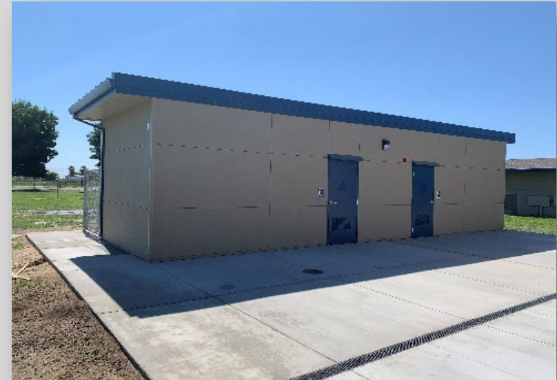
AFTER - INDIANOLA RESTROOMS
