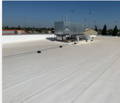
Selma High School Gym / Locker Reroofing Completed 02/2024 $931,122
