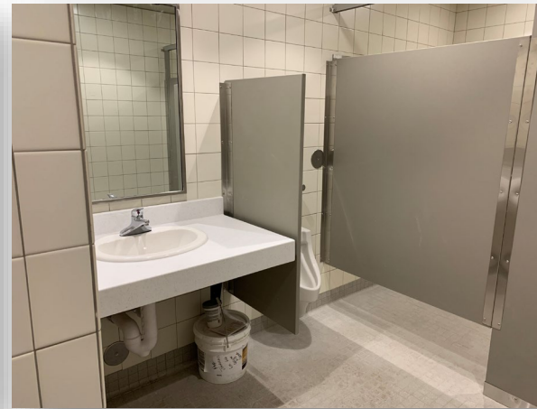
District office Restrooms
