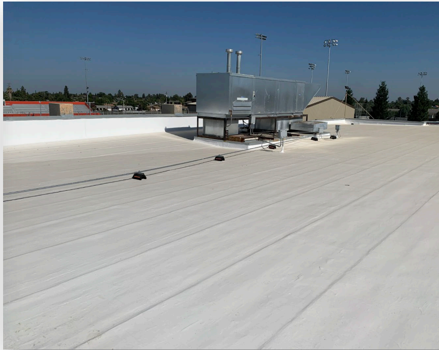
Selma High School Gym / Locker Reroofing
