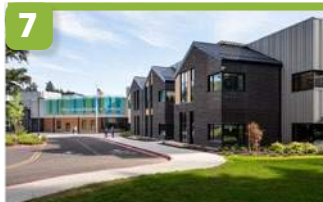
7 River Grove Elementary School
