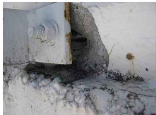
Spalling at Ladder Anchorage
