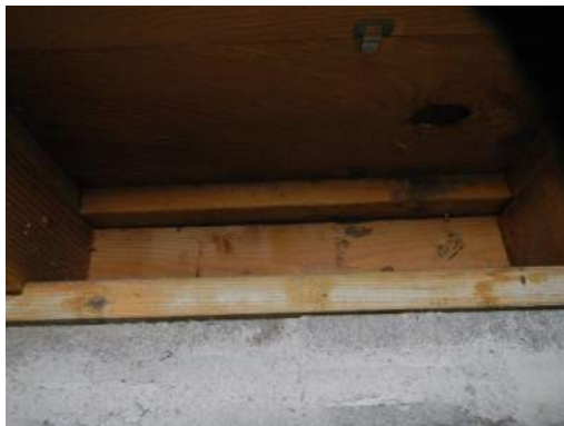
Inadequate Diaphragm to Wall Connection
