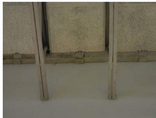
Inadequate Diaphragm Connection
