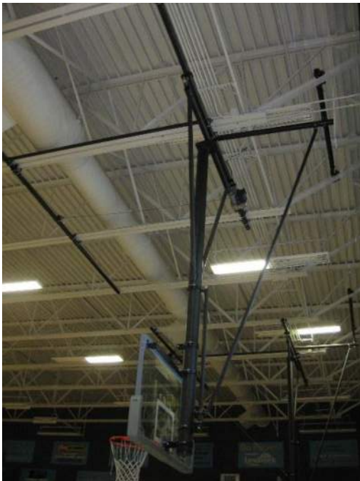
Backboard Braced to bottom of Truss – Deficiency
