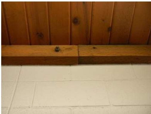
Missing Bolt in Ledger
