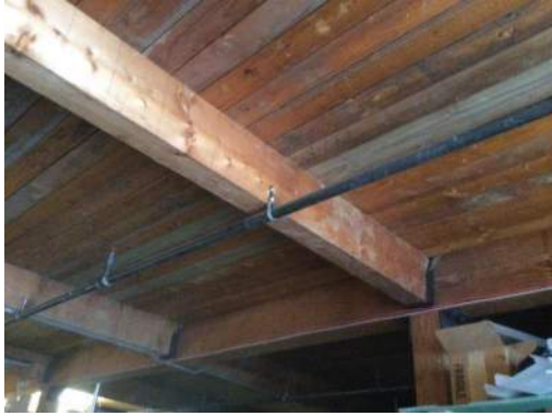
Remove Straight Sheathing
