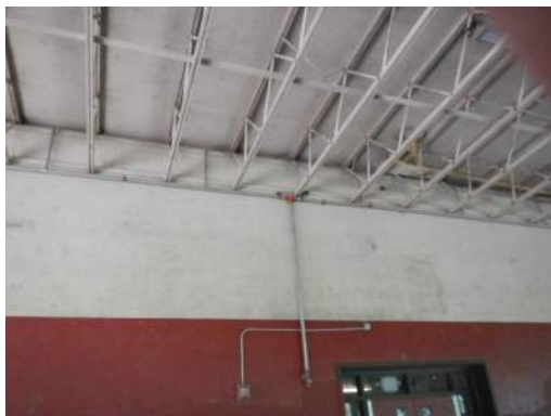
Inadequate Diaphragm Connection
