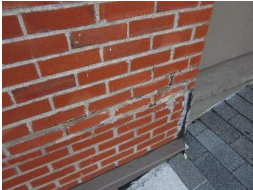
Brick Veneer Cracking
