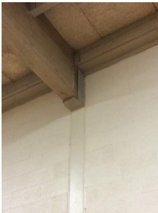
Inadequate Diaphragm Connection
