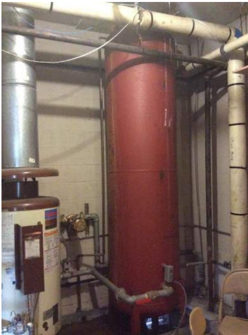
Tank to be Braced from Wall
