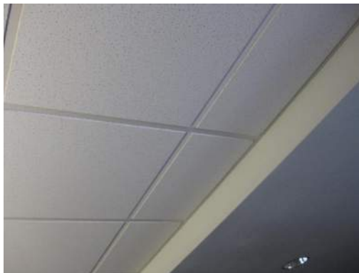
Ceiling Edge Clearance Deficient
