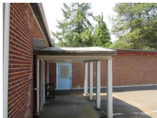
Unknown Lateral Connection Deflecting Side Entry Canopy
