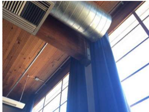
Lack of Seismic Connection & Beam Support
