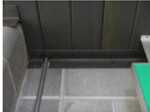
Missing Diaphragm Connection to Ledger
