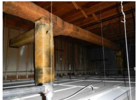
Unbraced Ceiling Tiles
