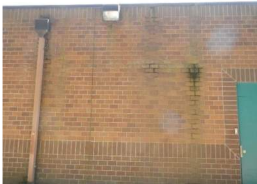
Brick Veneer Cracking
