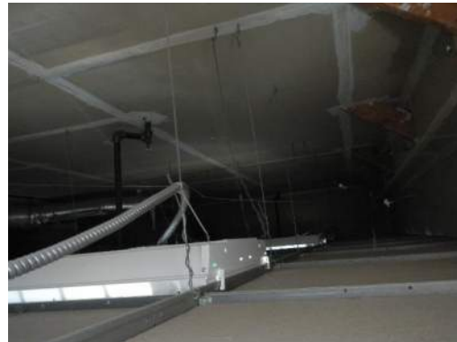
Unbraced Ceiling Tiles
