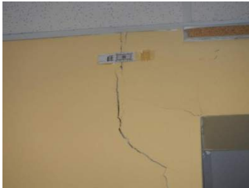
Cracks in Masonry Walls
