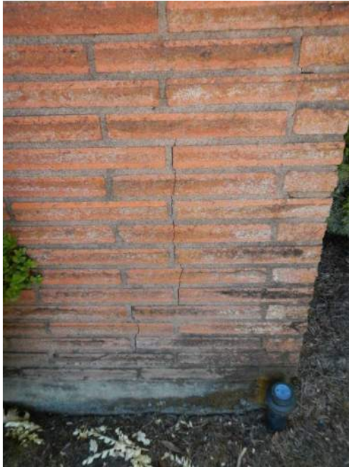
Cracking in Brick Veneer
