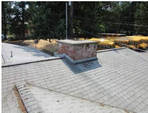
Unreinforced Brick Chimney
