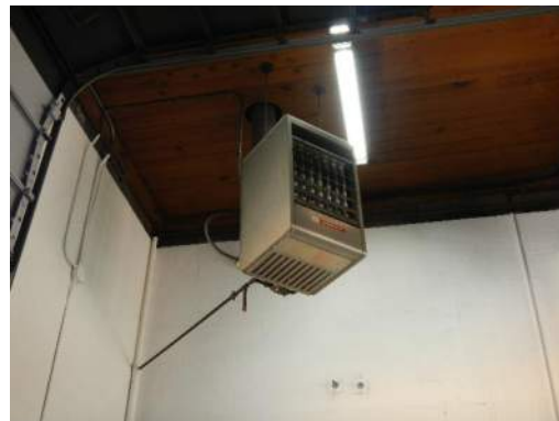
Unbraced Equipment
