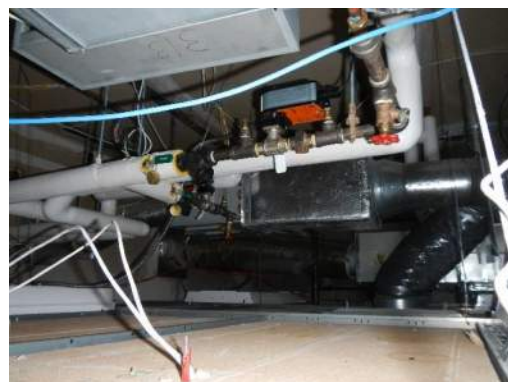
Unbraced Piping
