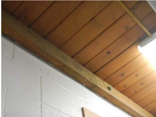
Inadequate Diaphragm Connection
