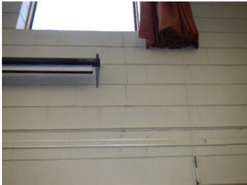
Crack in Masonry Wall
