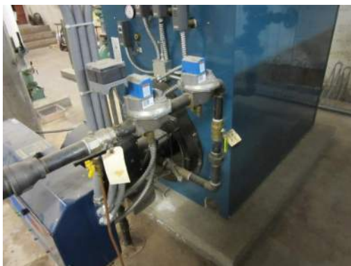
Hard Connected Gas Line
