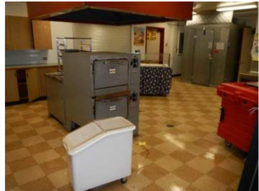
Unanchored Equipment in Kitchen
