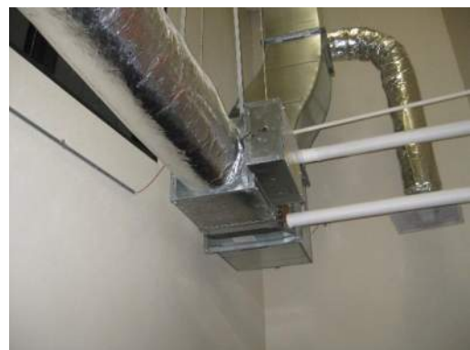
In-line Equipment Not Braced
