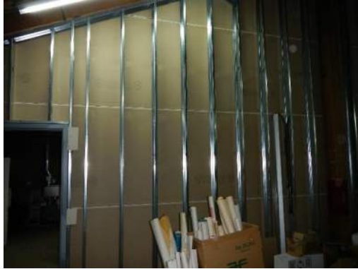
Wall Needs Blocking & Strapping
