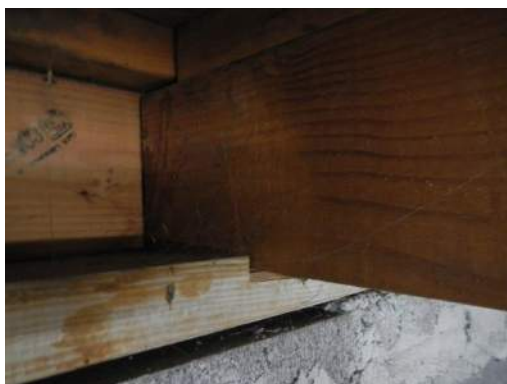
Inadequate Joist Connection to Wall
