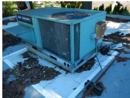
Inflexible MEP Connections
