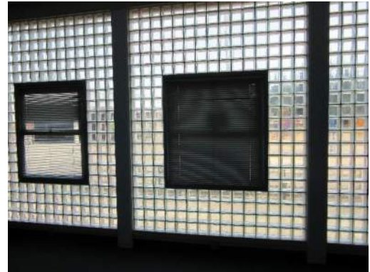
Unreinforced Glass Block Wall
