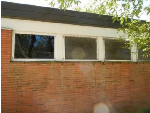
Water Damage in Brick Veneer
