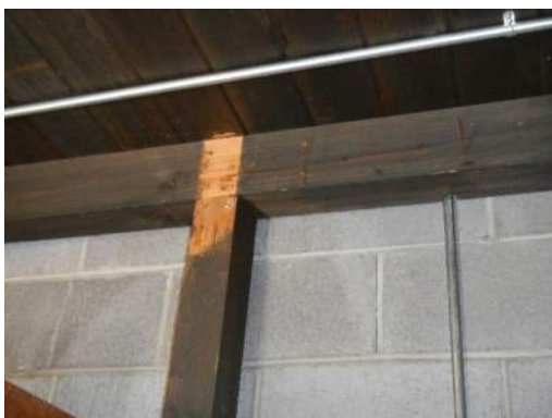
Missing Connection Hardware
