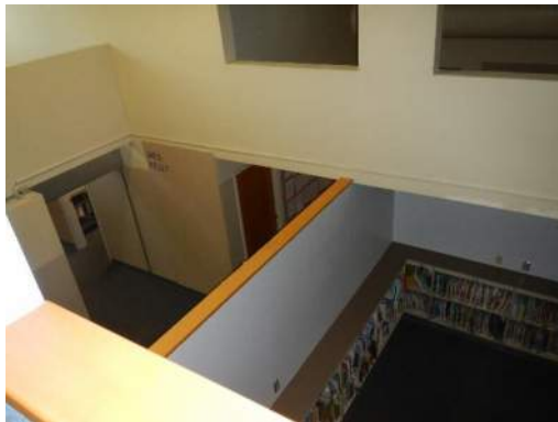
Unbraced Partial Height Walls
