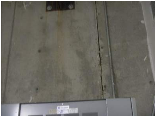
Cracks in Concrete Walls
