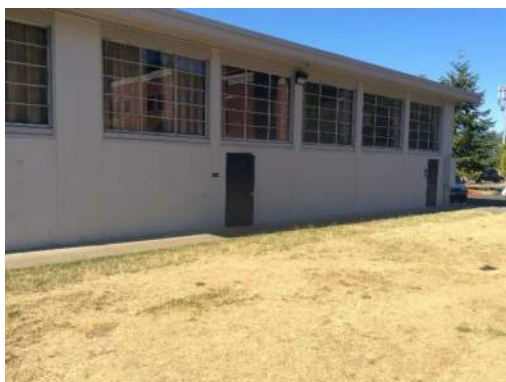
Lack of Lateral Support at Building End
