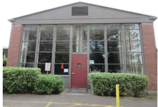
Lack of Lateral Support at Building End
