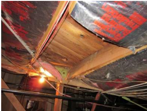
Plank Sheathing without Plywood
