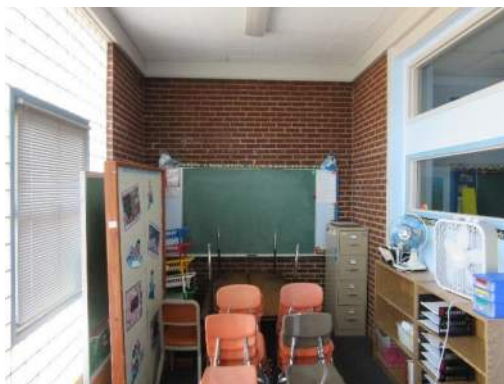
Unreinforced Brick Wall
