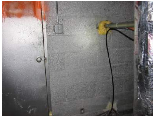
CMU Wall without Seismic Restraints
