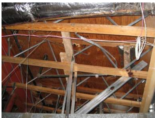
Unbraced Fire Suppression Piping
