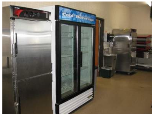
Unbraced Tall Refrigerator – Falling Hazard
