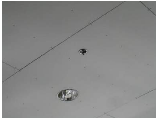
Sprinkler Head Clearance Not Adequate
