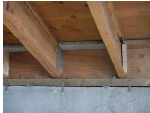
Inadequate Diaphragm Connection
