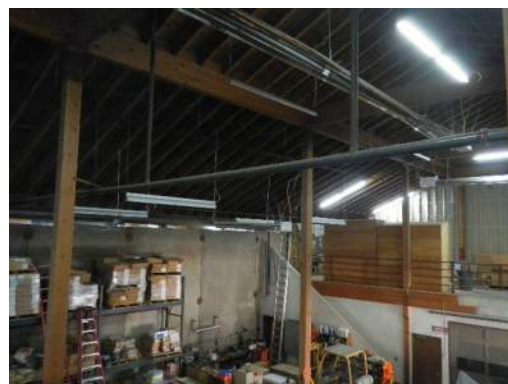
Unbraced Piping
