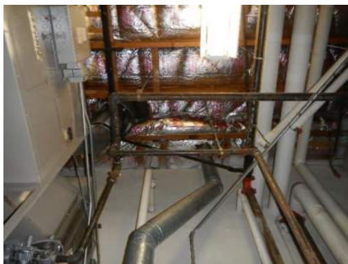
Unbraced Pipes
