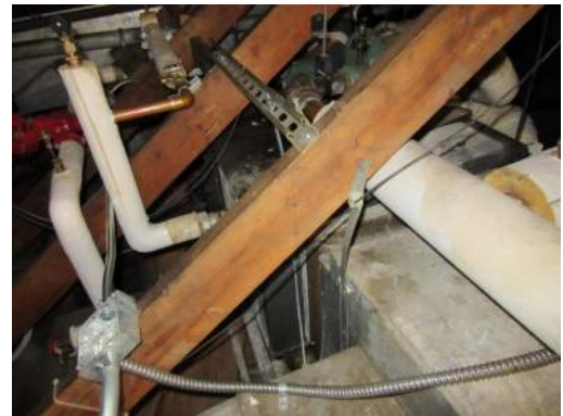
Hard Connected Gas Line & Fall Prone Equipment
