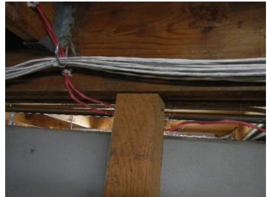
Post to Girder Inadequate Connection
