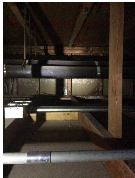
Unbraced Piping
