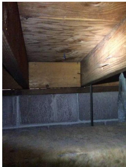
Inadequate Joist Connection
