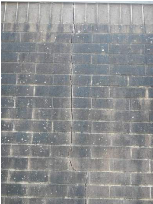
Cracking at Exterior Veneer
