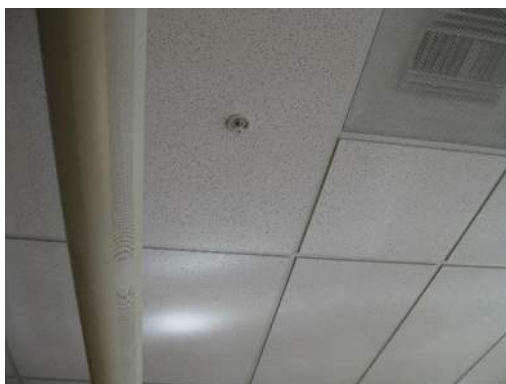
Sprinkler Head Clearance Deficient
