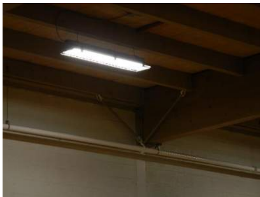
Cross-Grain Bending Induced in Joist
