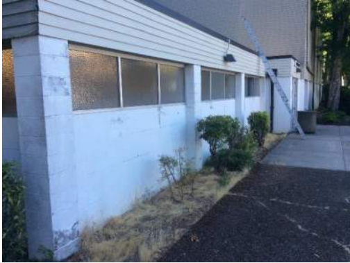
Lack of Lateral Support at Building Side
