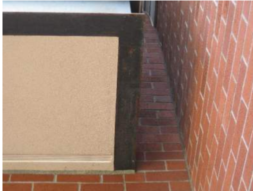
Rust on Pop-out Steel Framing
