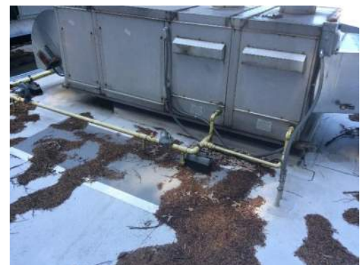
Hard Connected Gas Line
