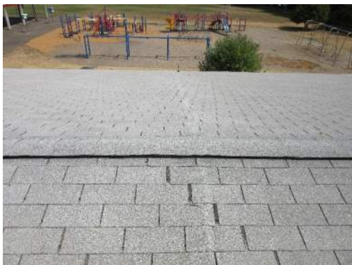
Roof Deflection at Building Joint
