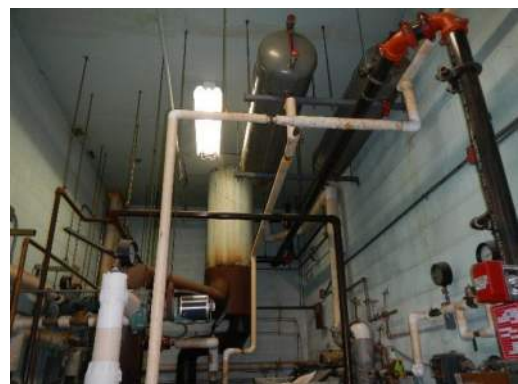
Unbraced Piping
