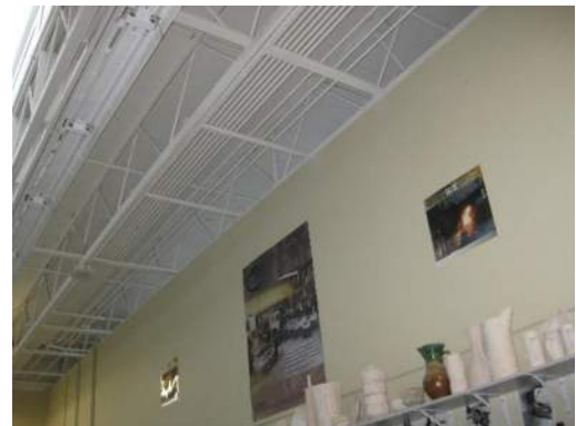
Partition Wall Attached to Unbraced Bottom Truss Chord
