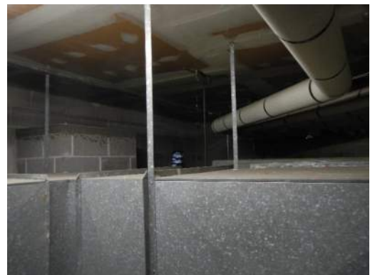
Unbraced Piping
