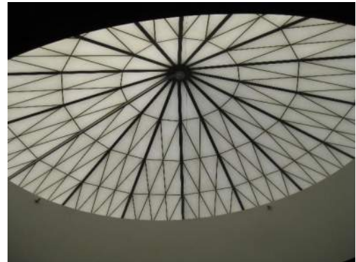
Overhead Glazing Falling Hazard
