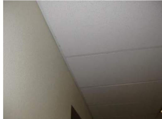
Ceiling Edge Clearance Deficient
