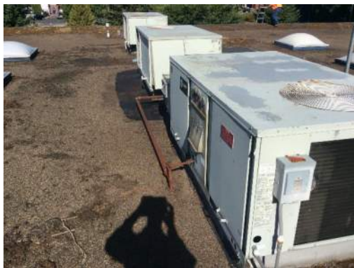
Hard Connected Gas Lines
