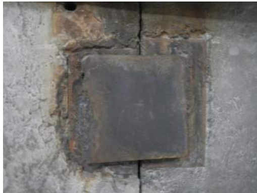
Corrosion in Panel Connections
