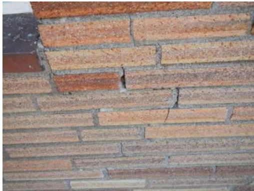
Cracking in Brick Veneer
