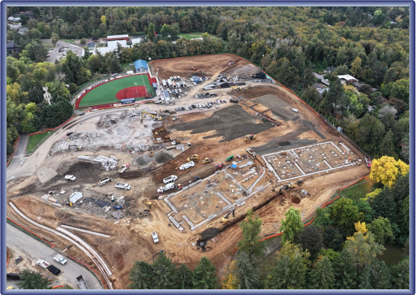
LOMS Construction Site
