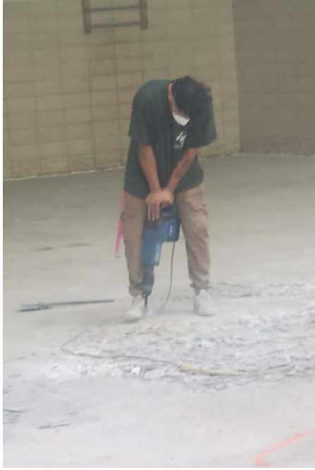
Above: Area of old floor base being removed (L); new concrete poured to level floor (R)
