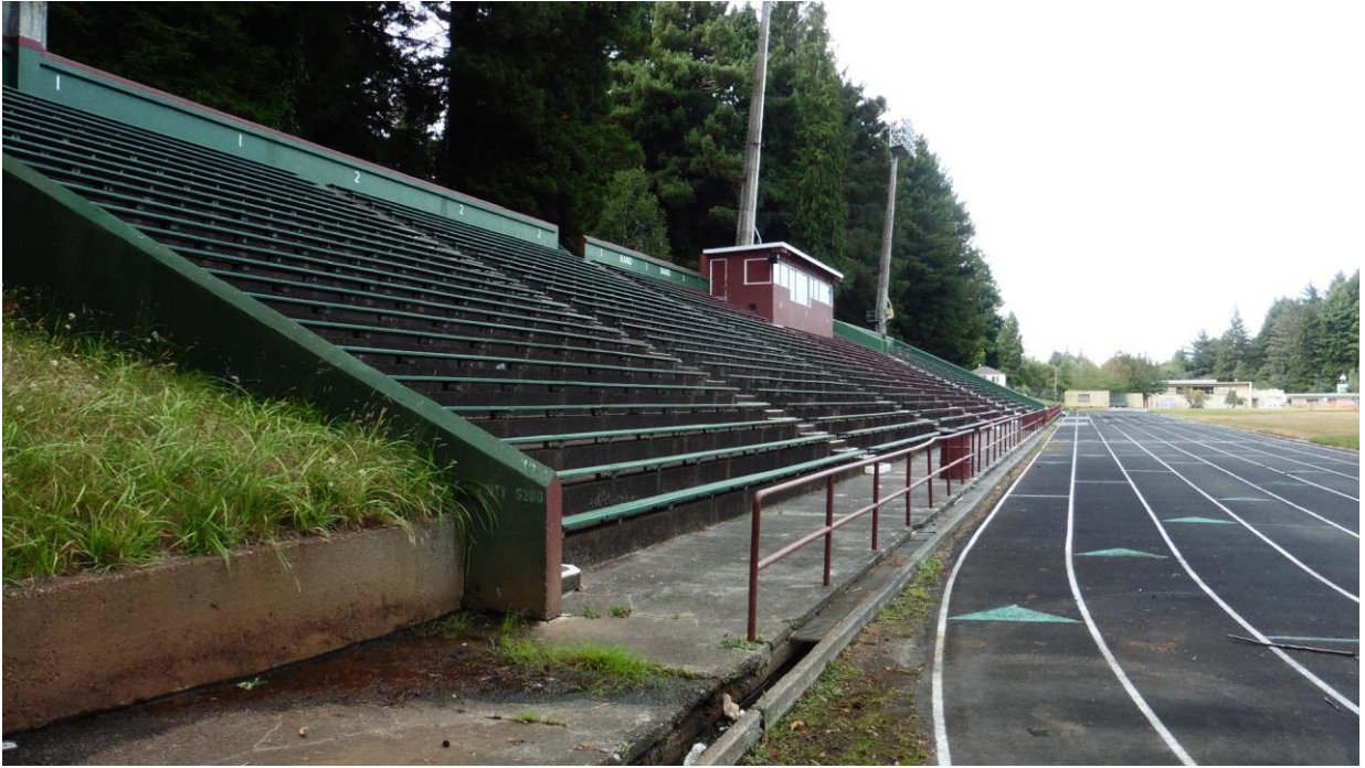
Photo 1: Looking north along track and western edge of football field from TP40 location. Note water weeping from concrete retaining wall near TP40. Photo taken September 21, 2020.
