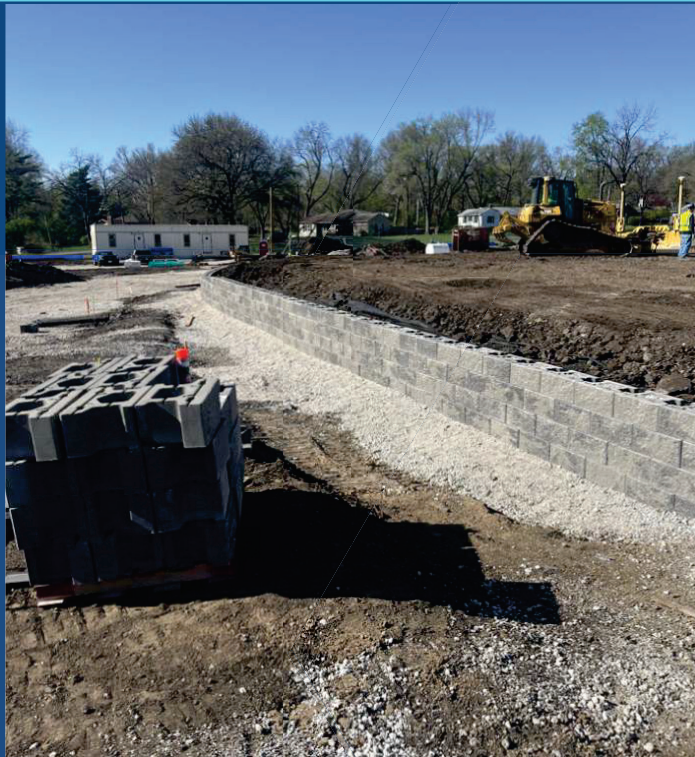
Retaining Wall Install
