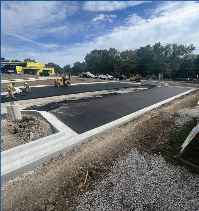
South Lot Asphalt Install
