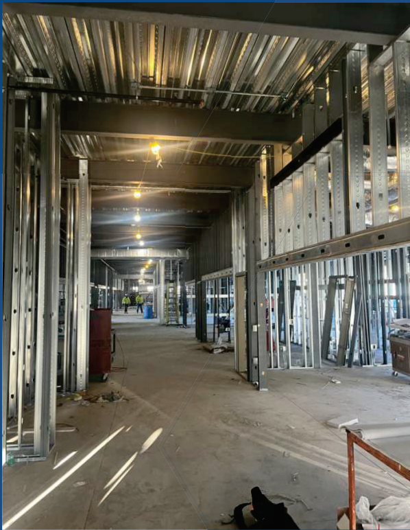
First Floor Interior Framing
