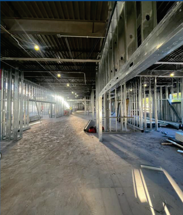
Second Floor Interior Framing
