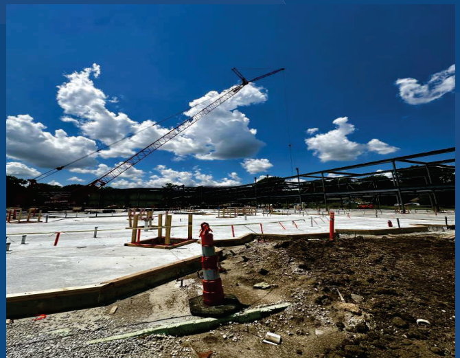
Completed Concrete Slab
