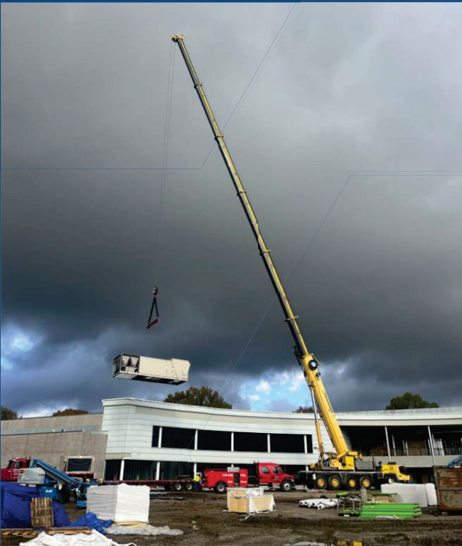
RTU Installation
