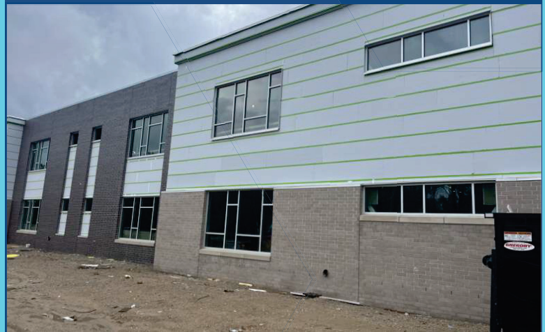
Exterior Glazing & Panel Install
