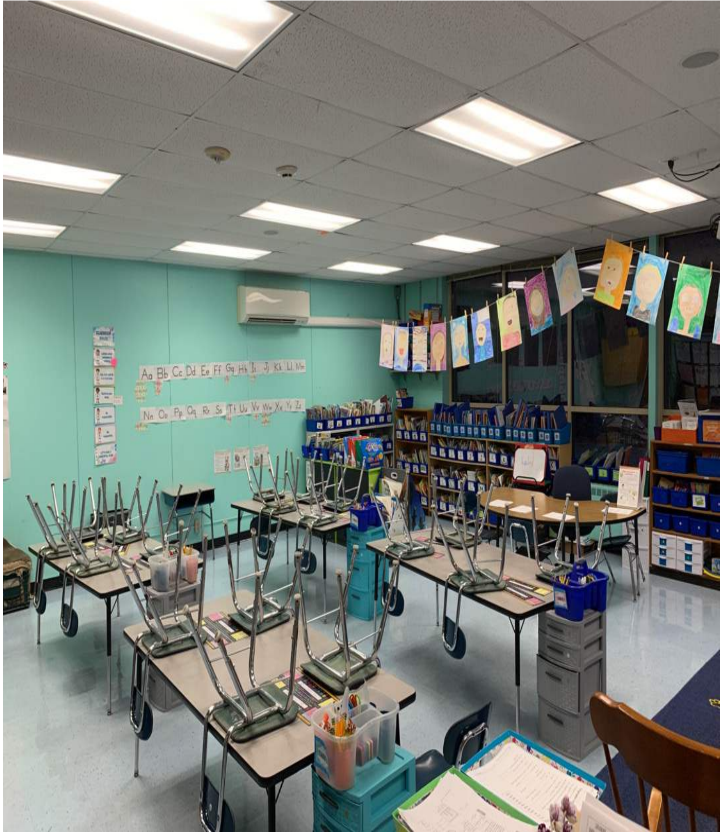
Room 18 – Area of Concern
