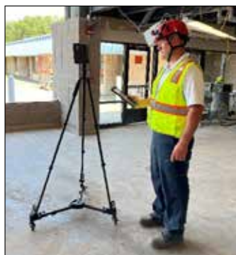
Fire Marshal York utilizes the DTFM's Matterport Pro3 camera at the Windermere Elementary construction site to capture the progress.
