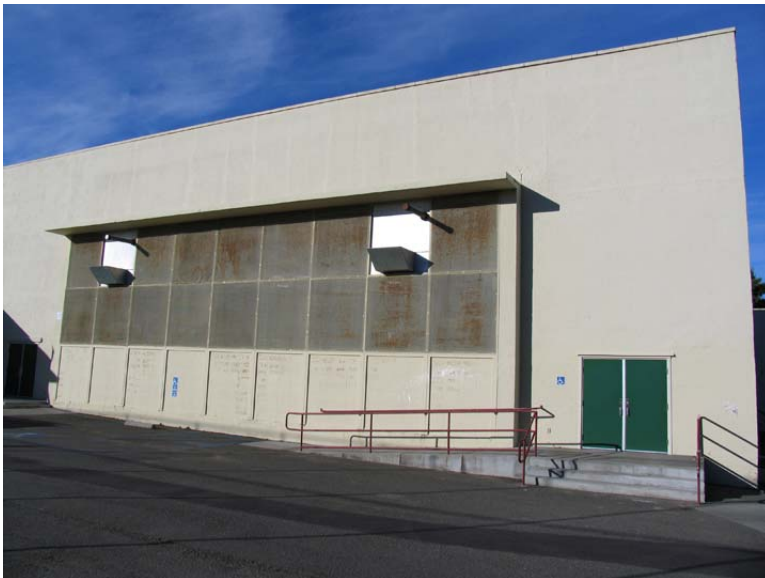
South elevation of natatorium portion, windows have received infill panels (lowest row), metal screens, and mechanical ventilation units, 1/4/06
