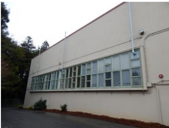
Figure 10: Typical double row of fixed and awning windows within a projecting concrete frame, as seen on the north façade, looking southeast.
