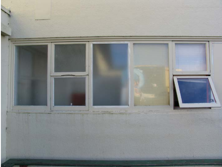
Window type - Wood fixed and stacked (two-high) awning windows aligned in continuous band and set in stepped frame (example located near secondary entry, north façade of girls' gym wing), 1/4/06
