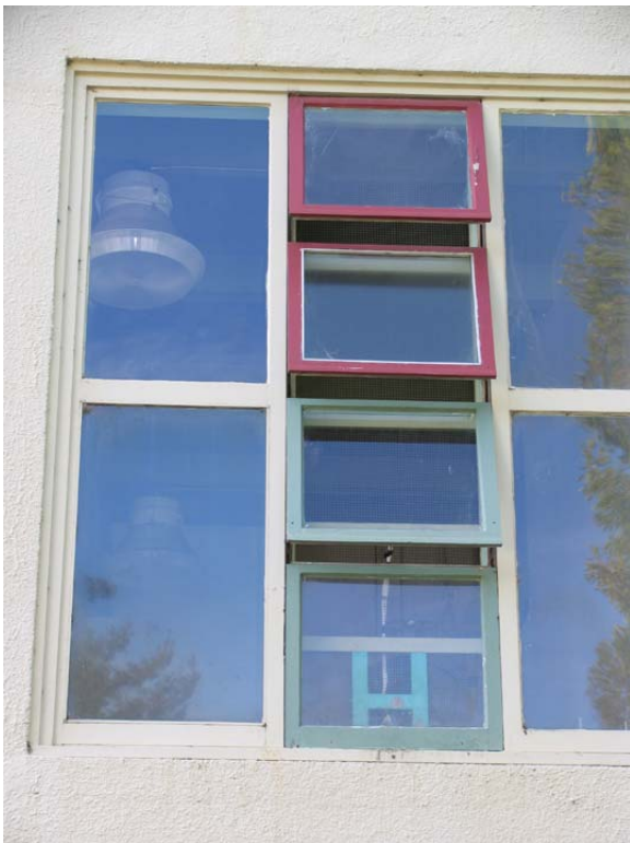
Window type – Wood fixed and stacked (four-high) awning windows aligned in continuous band and set in stepped frame (example located at north elevation), 1/4/06
