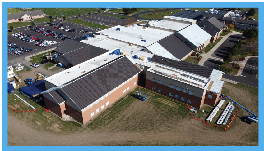
RVHS Metal and Low Slope Roof Installation
