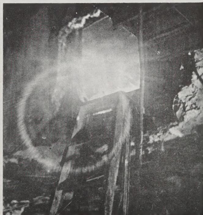
Bizarre shot captures the halo of light from welders' torches as workmen labor deep within the boiler.
