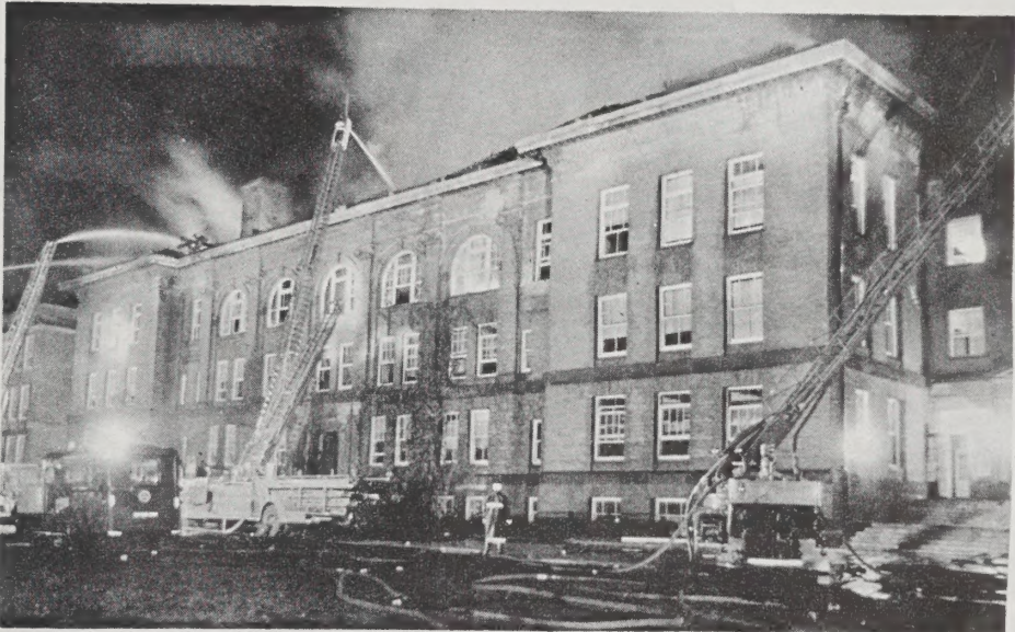
Aerial hoses shower Building B at climax of multi-million dollar disaster. (Boston Globe photo)
