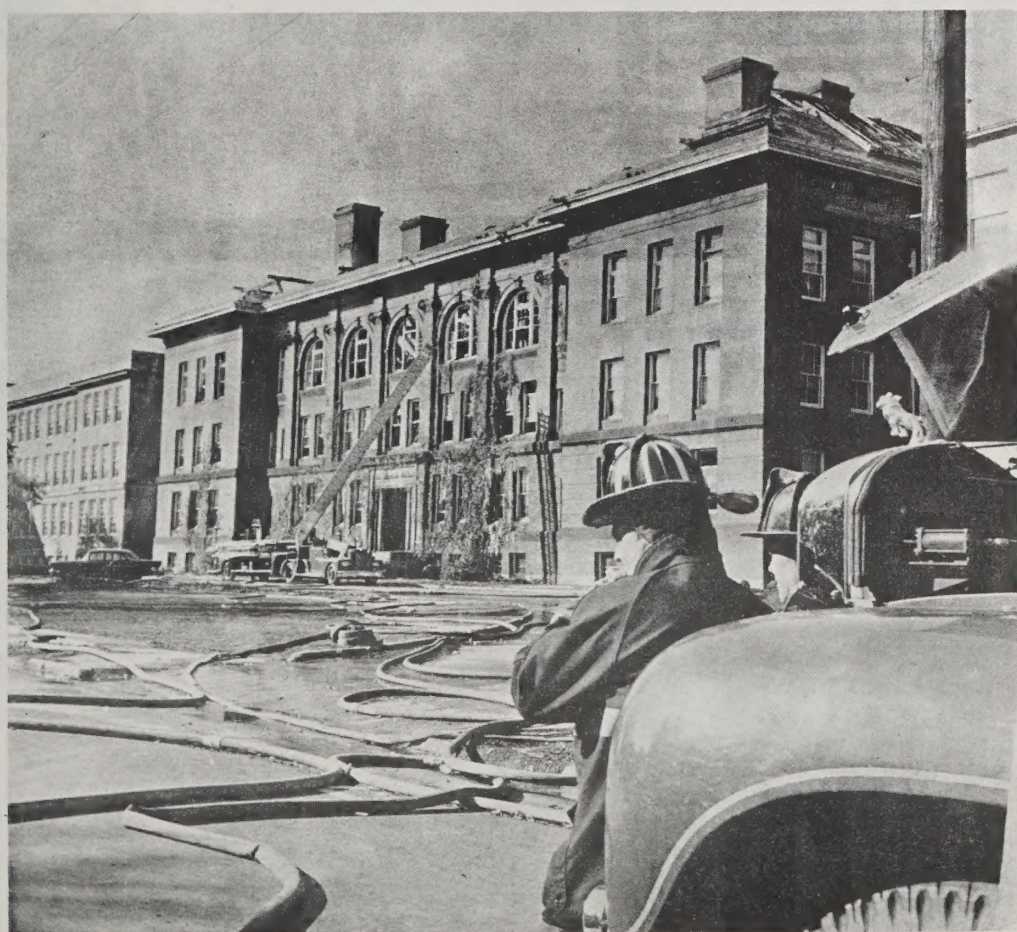
The aftermath. Still on the job 16 hours later, tired Medford firefighters stand numb in cold air trying to catch their second wind. Ladder truck rests against Science Office window as years of traditional ivy hangs against fire-gutted building.
