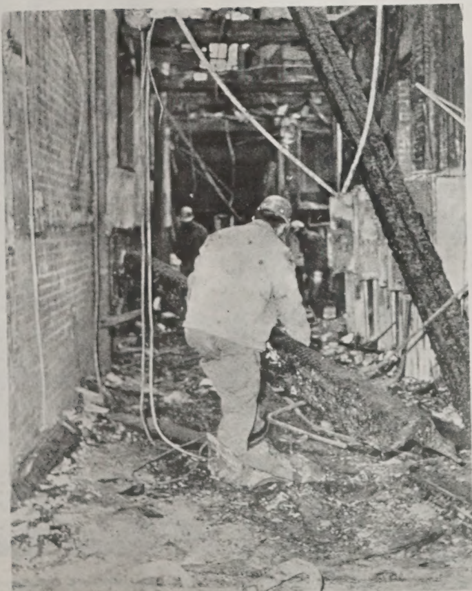
Workmen start tedious task of ripping down charred walls.
