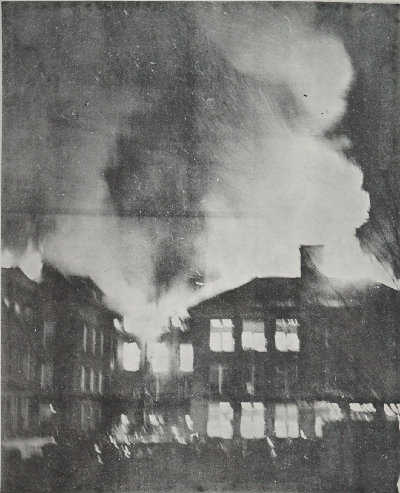
Hot air expulsion. Dramatic photo taken by Stanley, who was knocked backwards, causing his camera to jolt as the entire building flared up. Seven firefighters working on a ladder were rushed to the Lawrence Memorial Hospital with injuries received in this explosion.
