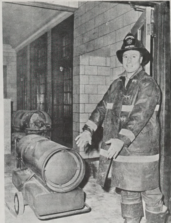
Firefighter R. Fiartrone warms his numbed fingers over one of the many portable heaters used to dry out Buildings A and D, the two saved wings.
