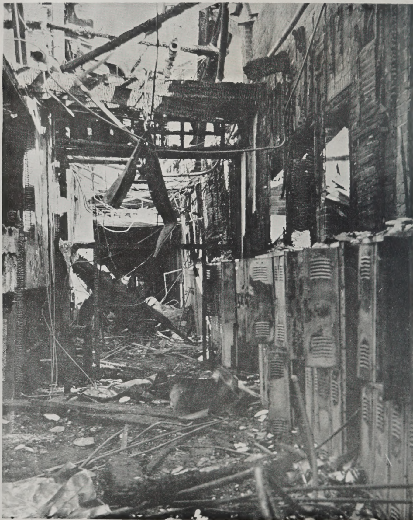
Scorched lockers, hanging beams, and massed rubble are all that remain of demolished 3rd floor.
