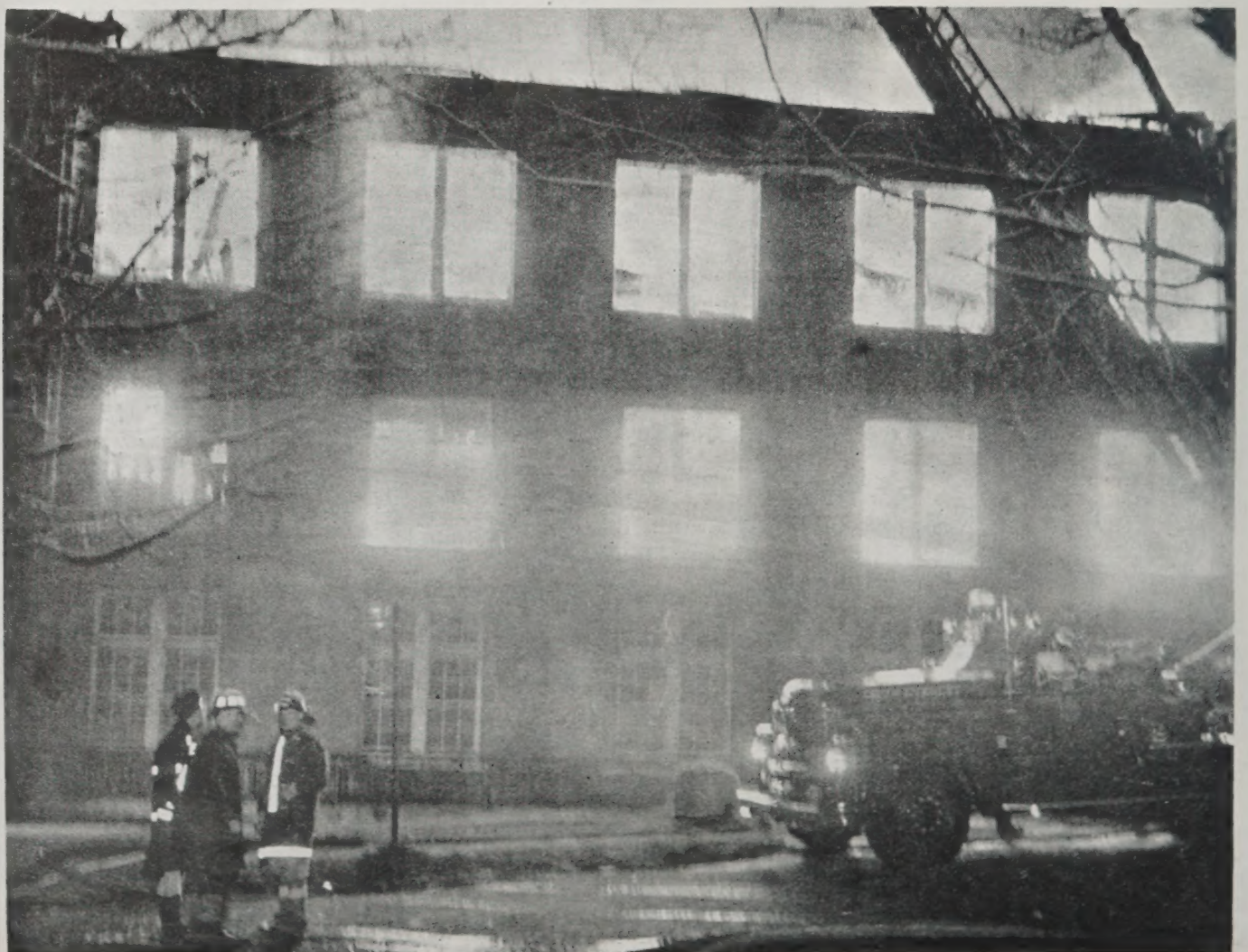
Every window ablaze, Everett firemen can do little to save historic building.
