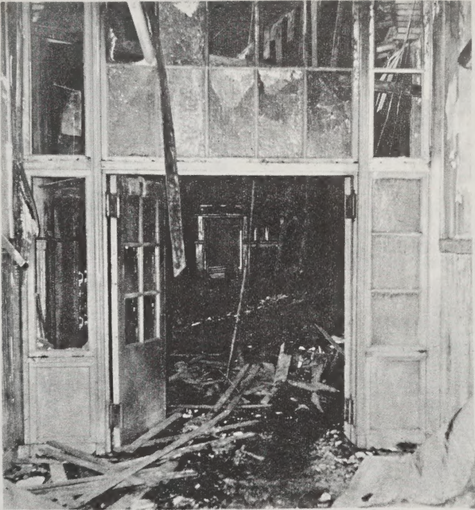
Medford's finest, Sgt. J. Humphrey, stands a lonely vigil before destroyed building. Inside, end of first floor crossover and Mr. Buckley's lab show extensive damage and fallen roof, while custodians and firemen work long hours to repair soaked boilers.
