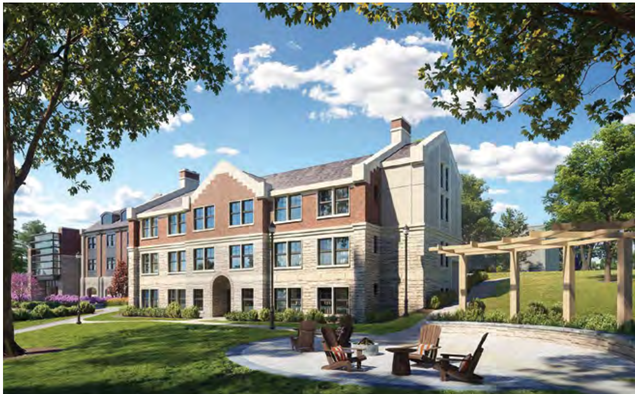
Also constructed in 1966 by architect Frank Perantoni '42 , Mason Hall, originally named "Mason House," pays homage to Marvin Garfield Mason, Blair's first track coach and English Department chair, who served the School for 41 years.
