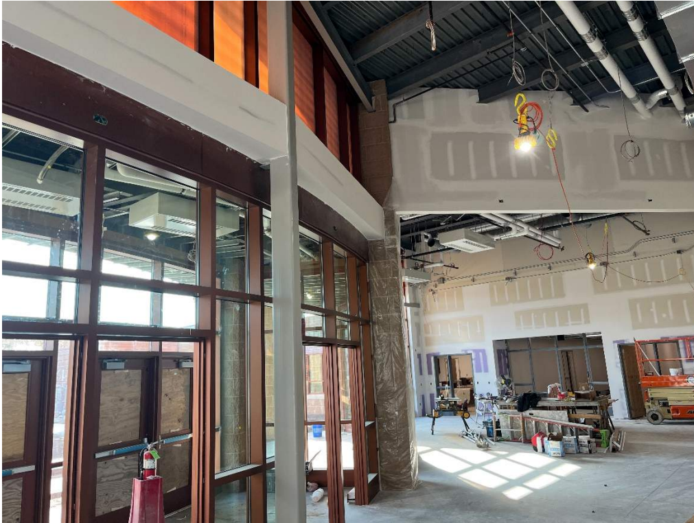
Segment D Radius Entry – Drywall Taping in-Progress
