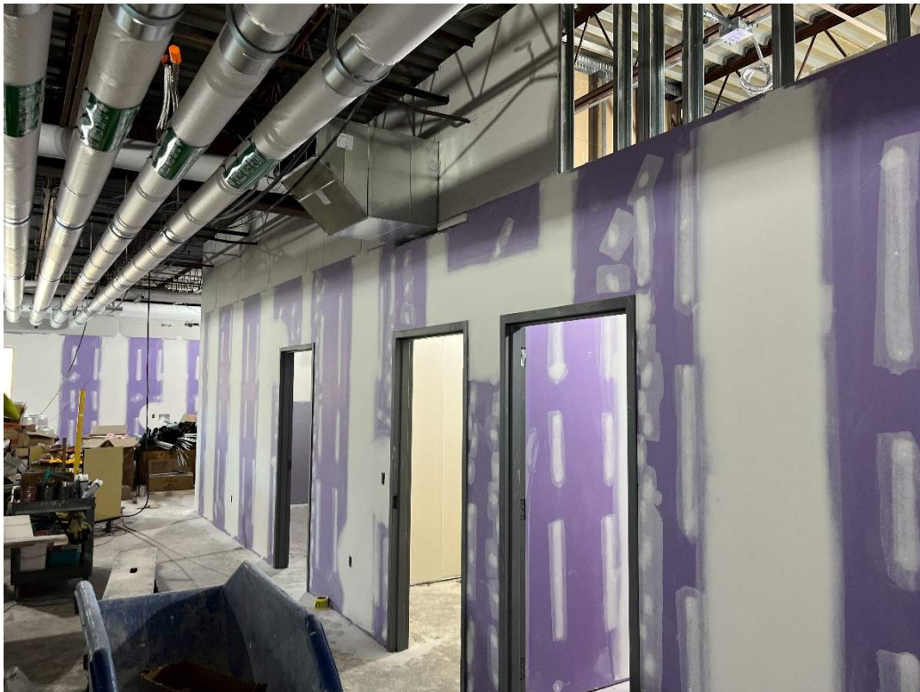
Segment F – ID Room Drywall Taping/Interior Painting in-progress.
