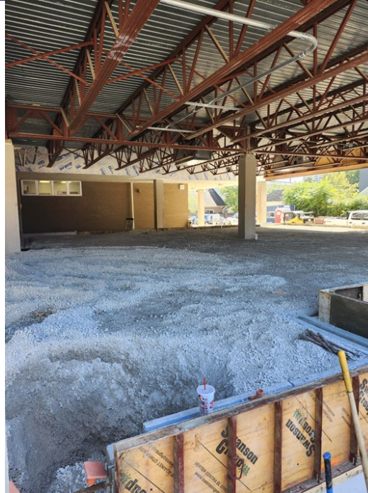
Backfill of Building Pad
