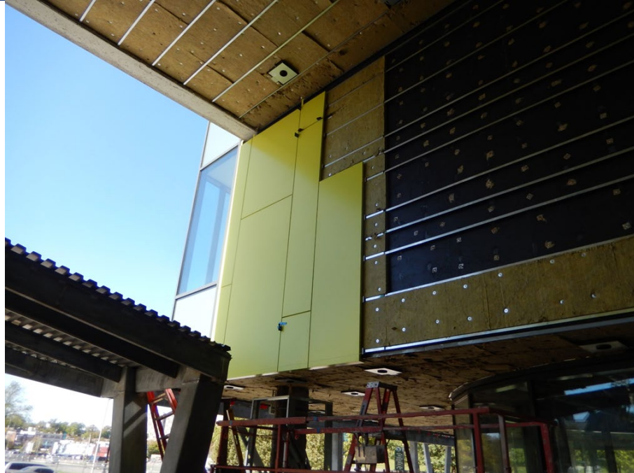
View of Composite Metal Panel at Main Entry
