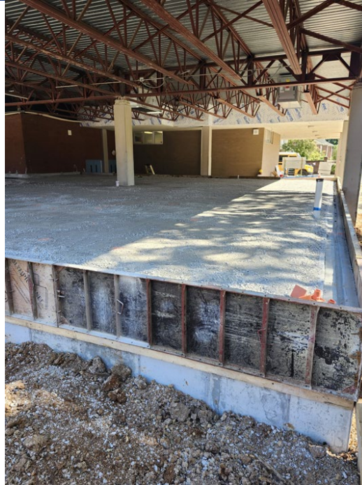
Backfill of Building Pad
