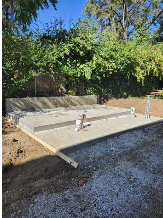
Poured Cooling Tower Pad
